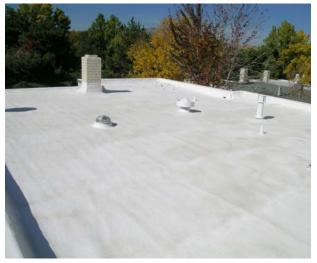
Light coloured roofs have a high solar reflectance, which reduces energy cost and reduces urban heat island effect.
