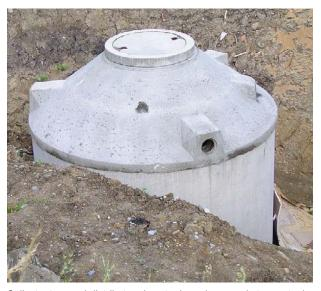
Collect, store and distribute rainwater in underground storage tanks.
