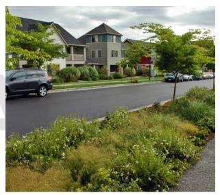
Local Road with a bioswale in the right-of-way to assist with run-off and infiltration.
