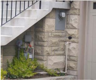
Utility meters are built into the facade of the exterior wall of the house, or to the side of the house with some landscaping in order to screen the meters from public view.
