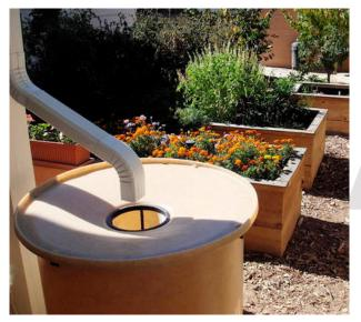
Rain barrels are storage tanks for temporarily holding stormwater. A house can have more than one rain barrel, and barrels vary in size and features.
