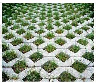
Permeable pavers to support on-site stormwater infiltration.
