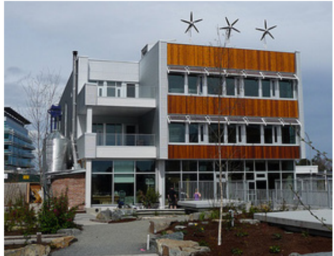
Wind turbines on the roof of an office building.
