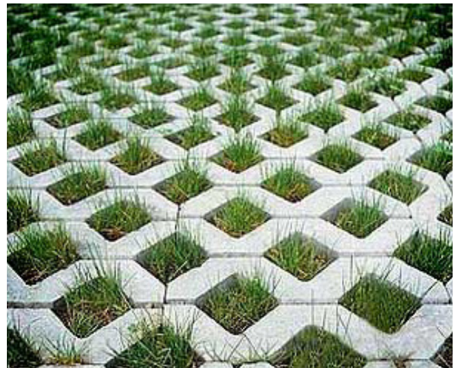
Permeable pavers to support on site stormwater infiltration.
