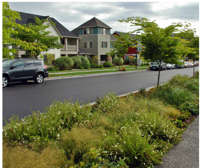
Local Road with a bioswale in the right-of-way to assist with run-off and infiltration.
