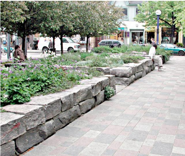
Light coloured pavers assist with the reduction of heat island effect.
