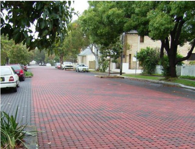
Example of the use of permeable paving material on a road.
