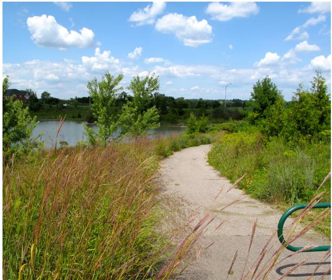
Trail designed using permeable materials.
