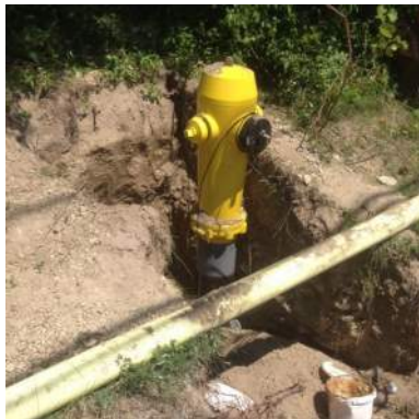
Installation of Hydrants
