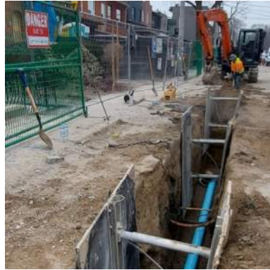
Open Cut Installation - Road
