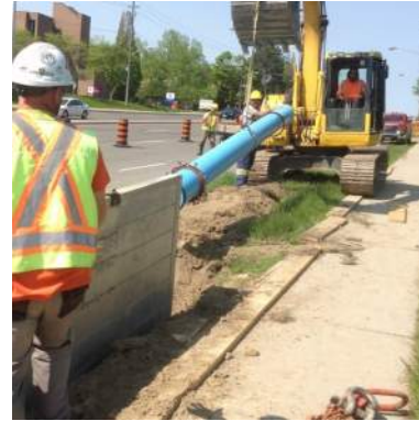
Open Cut Installation - Boulevard
