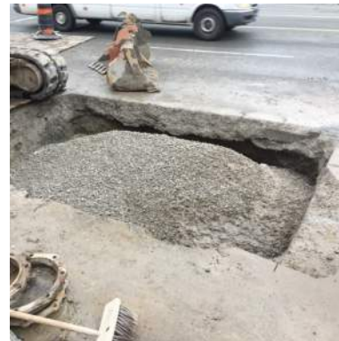
Trench Backfill
