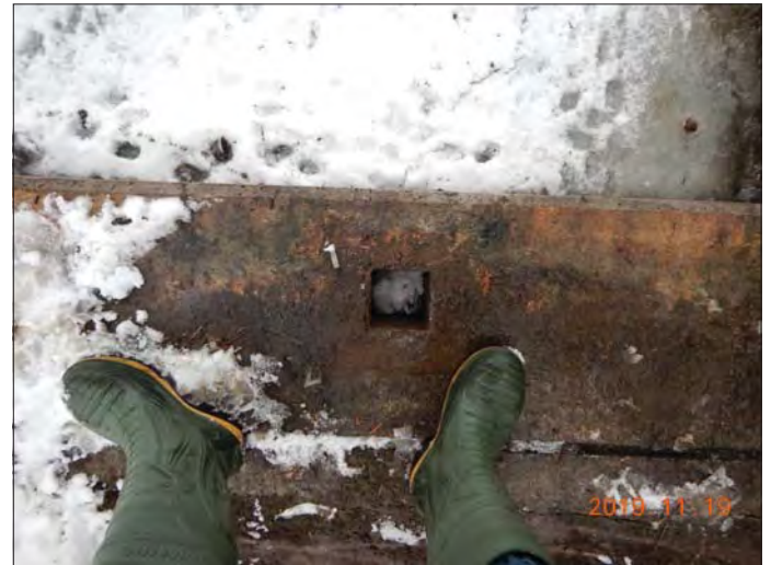
Photo 2735 - Sept 19, 2019 Pefferlaw Dam Flashboard Post Hole (Typical)
