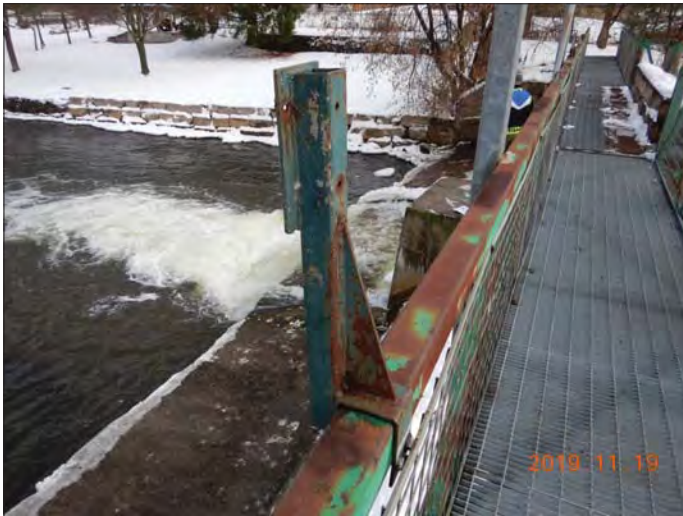
Photo 2790 - Sept 19, 2019 Pefferlaw Dam Remnants of Fish Ladder Bracket
