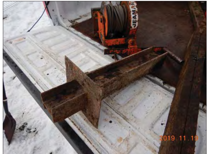
Photo 2856 - Sept 19, 2019 Pefferlaw Dam Typical Flashboard Post
