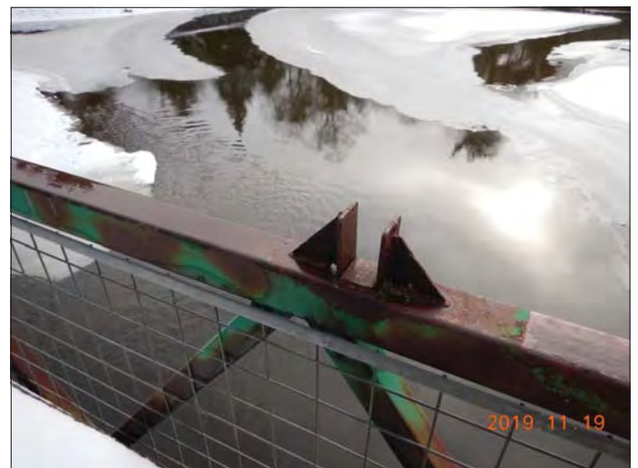
Photo 2796 - Sept 19, 2019 Pefferlaw Dam Winch Mounting Bar Bracket, Upstream Left
