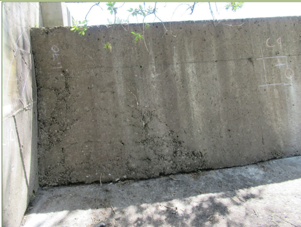
Photo P18 East Weir, North Elevation (cracks, spall and honeycombing)
