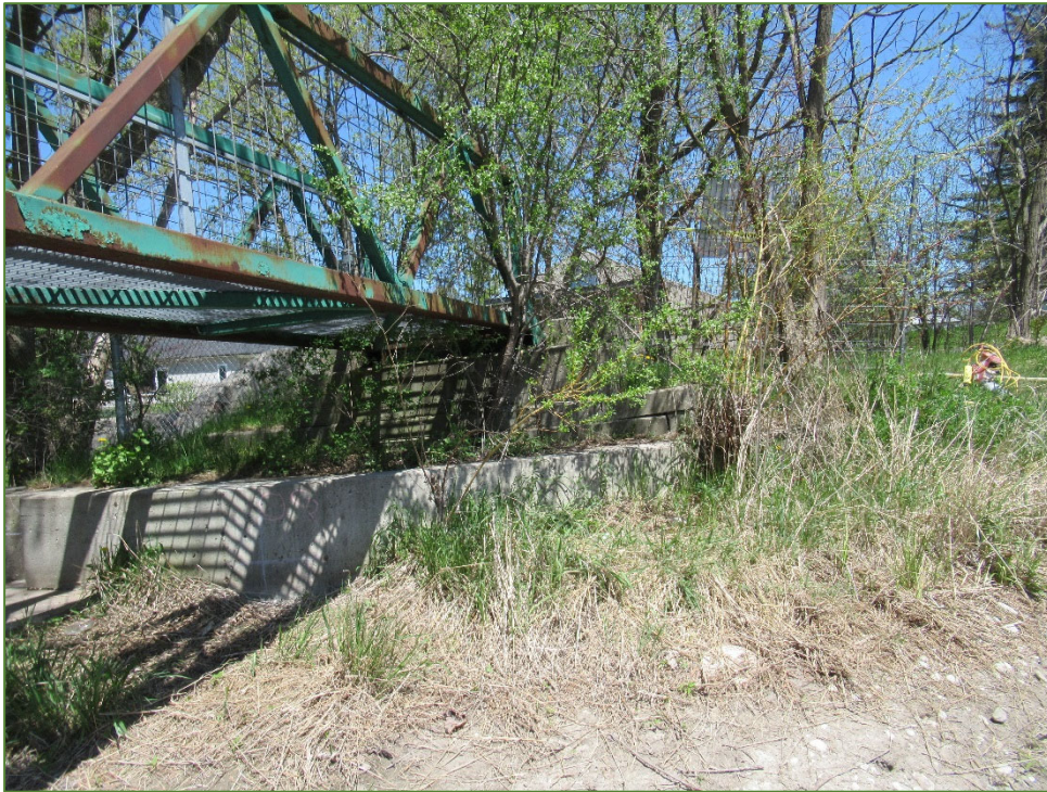
Photo P5 East Abutment and Retaining Wall (fair to poor condition – cracks, spall, delamination and light to severe scaling)
