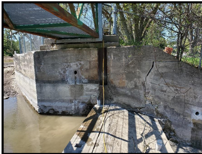
Photo 4 – West Abutment, Erosion at Waterline and Wide Vertical Cracking
