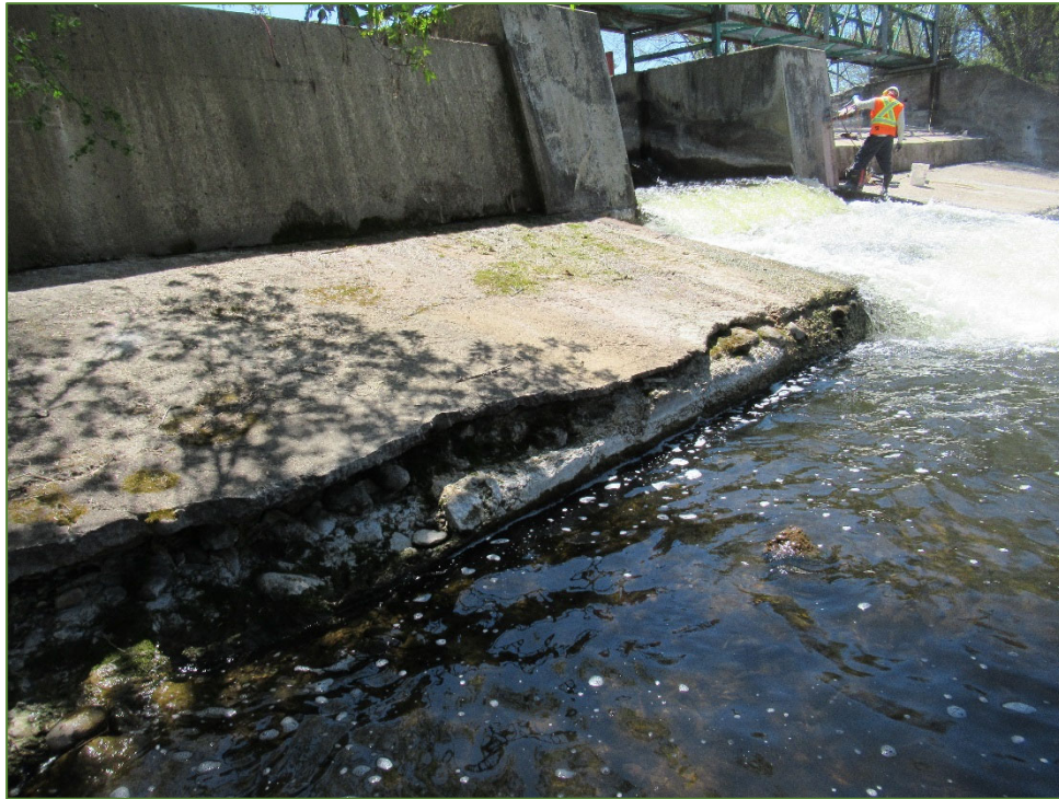
Photo P17 East Weir and Apron Slab, North Elevation (spall, delamination and medium scaling)
