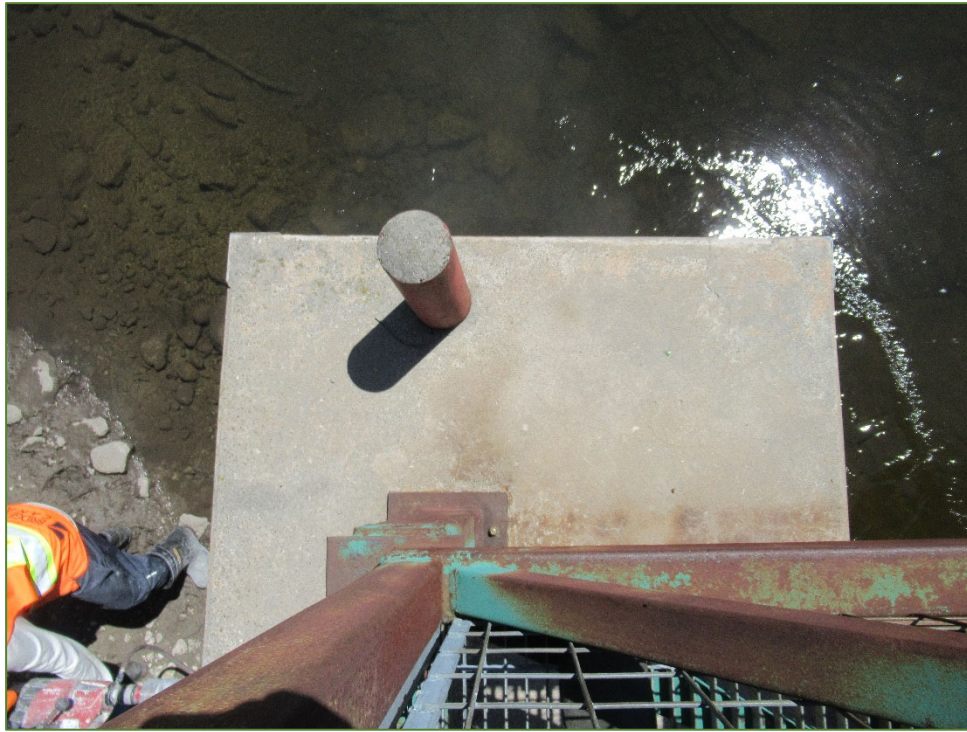
Photo P35 East Pier – Top Face (cracks and staining)
