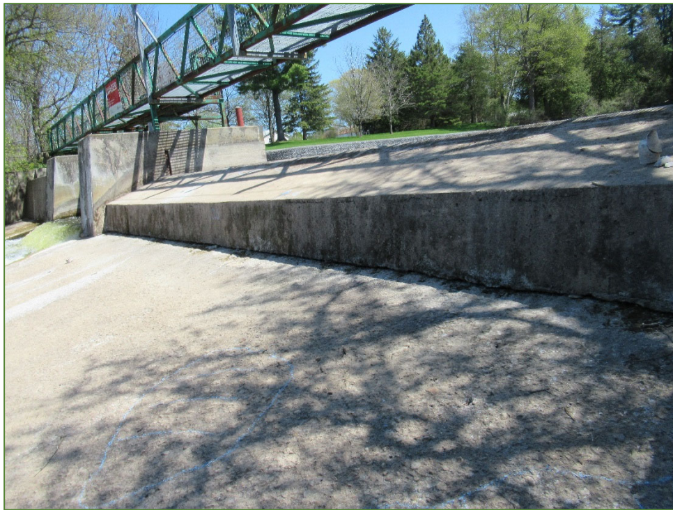
Photo P29 West Weir and Apron Slab – North Elevation (spall, delamination and medium scaling) note, undermining
