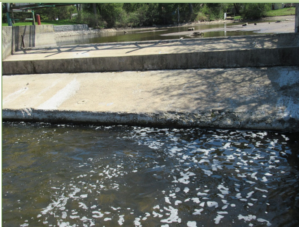
Photo P30 West Weir and Apron Slab – North Elevation (spall and medium scaling)
