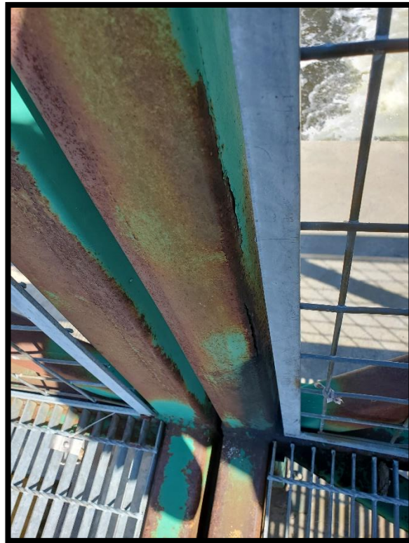
Photo 23 – Vertical HSS at Operational Span, Wide Cracks in Steel (1)
