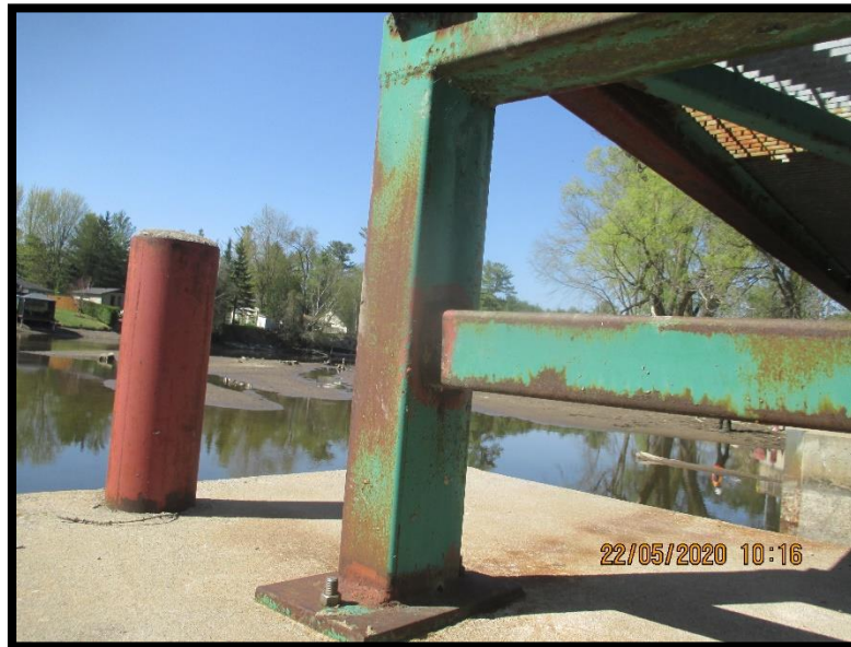
Photo 11 – HSS Support at West Pier, Loss of Protective Coating and Light Corrosion (Typ.)
