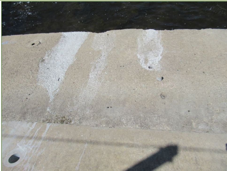
Photo P24 West Apron Slab Plan (spall and medium scaling)
