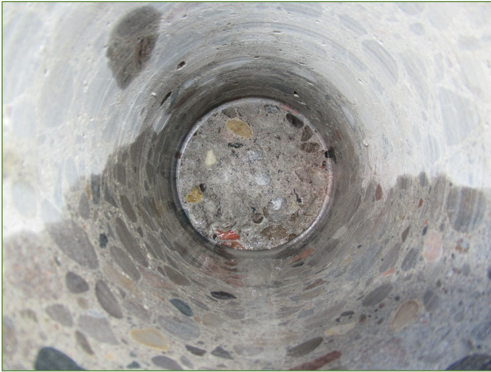
Photo P49 Typical Condition of Inside Core – C7
