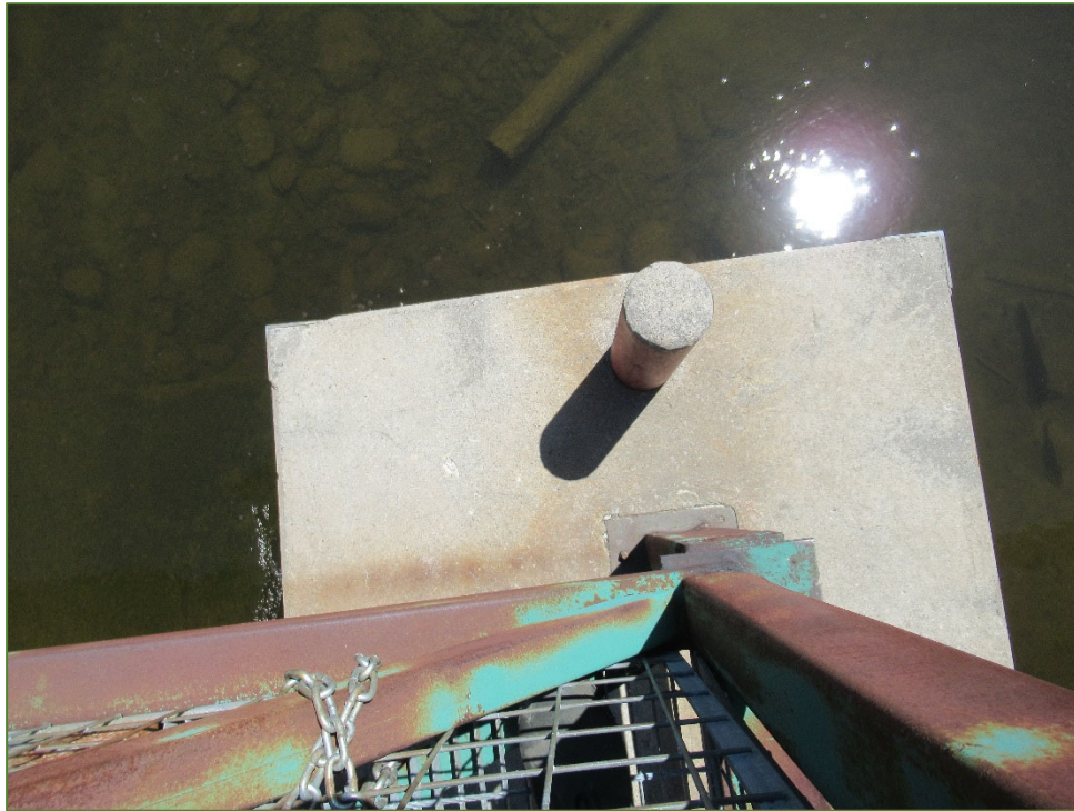
Photo P41 West Pier – Top Face (light scaling)
