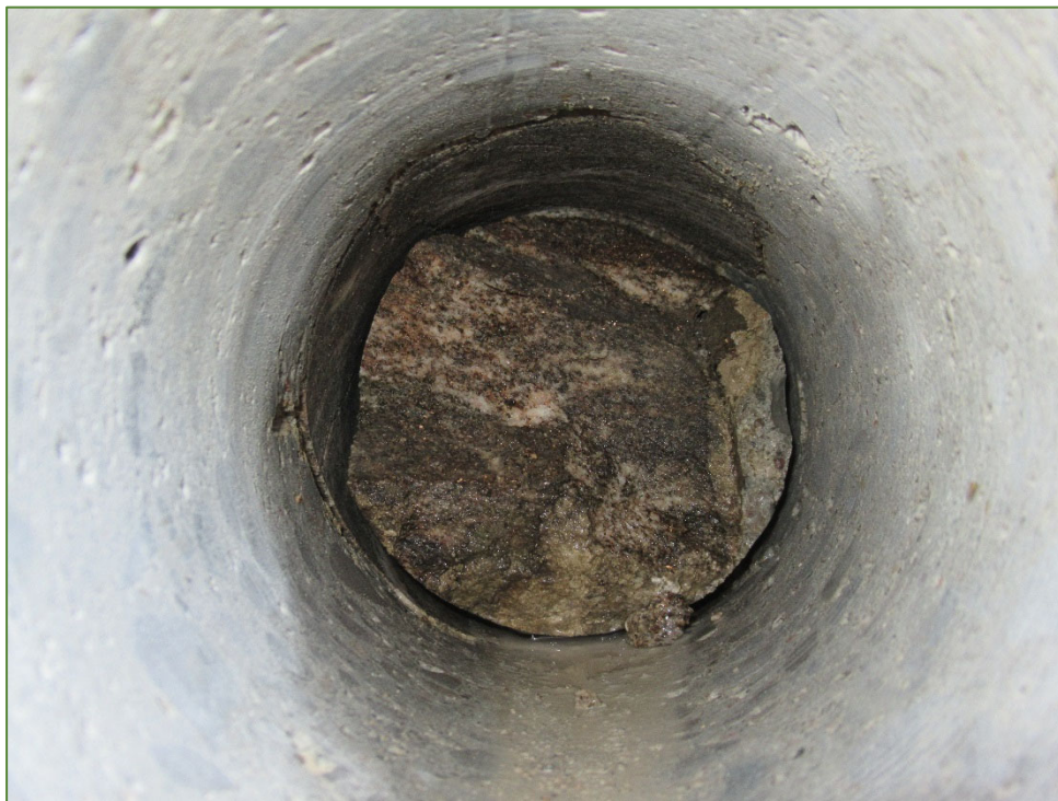
Photo P46 Typical Condition of Inside Core – C1 (delamination)
