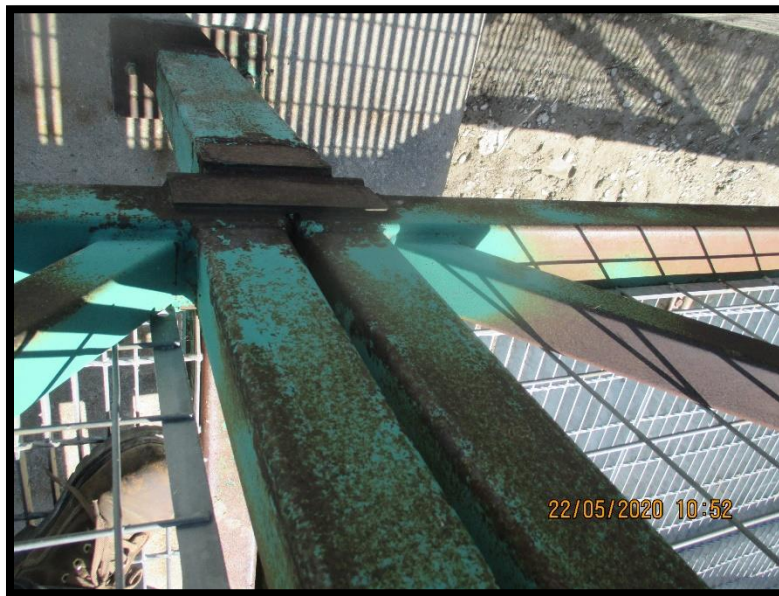
Photo 14 – Joint Between Operational and East Span, Loss of Protective Coating and Light to Moderate Corrosion (Typ.)
