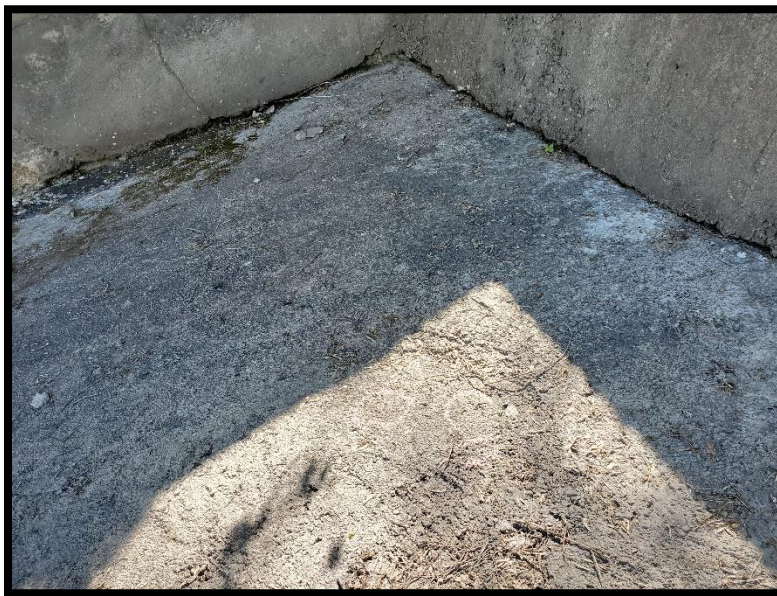
Photo 20 – East Concrete Apron, Medium Scaling (Typ.)
