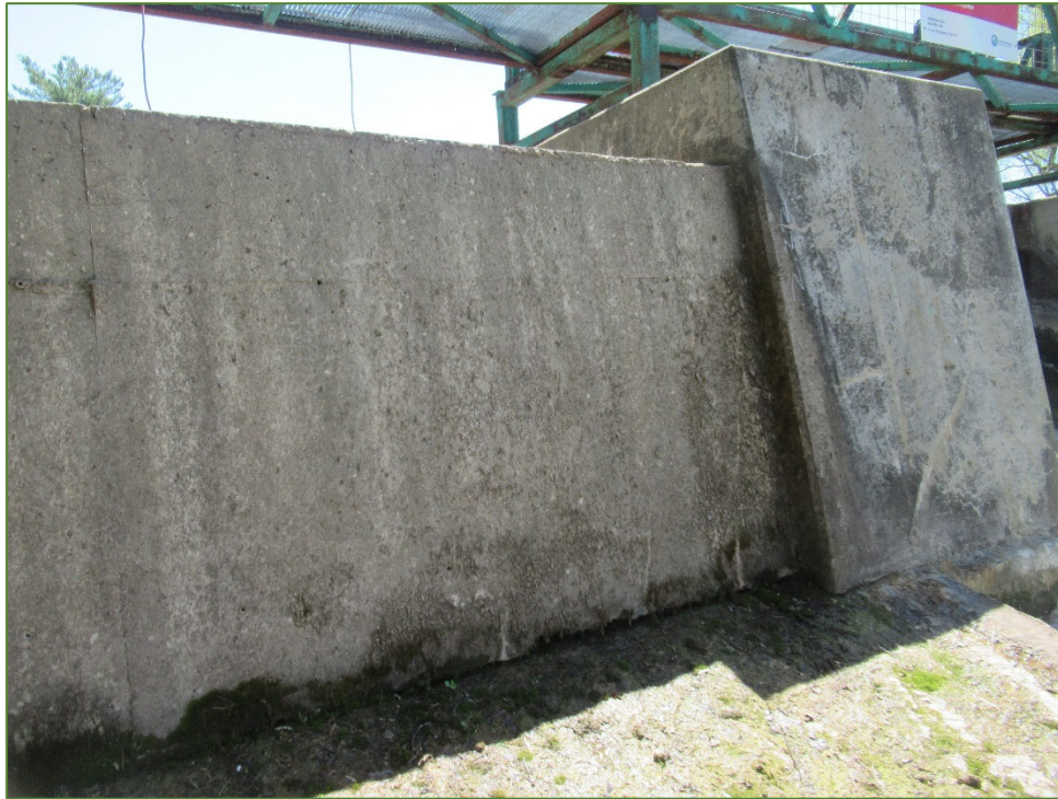
Photo P19 East Weir, North Elevation (light to medium scaling)
