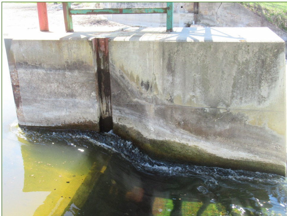
Photo P42 West Pier – East Face (fair to good condition – cracks, light scaling and wet stain)
