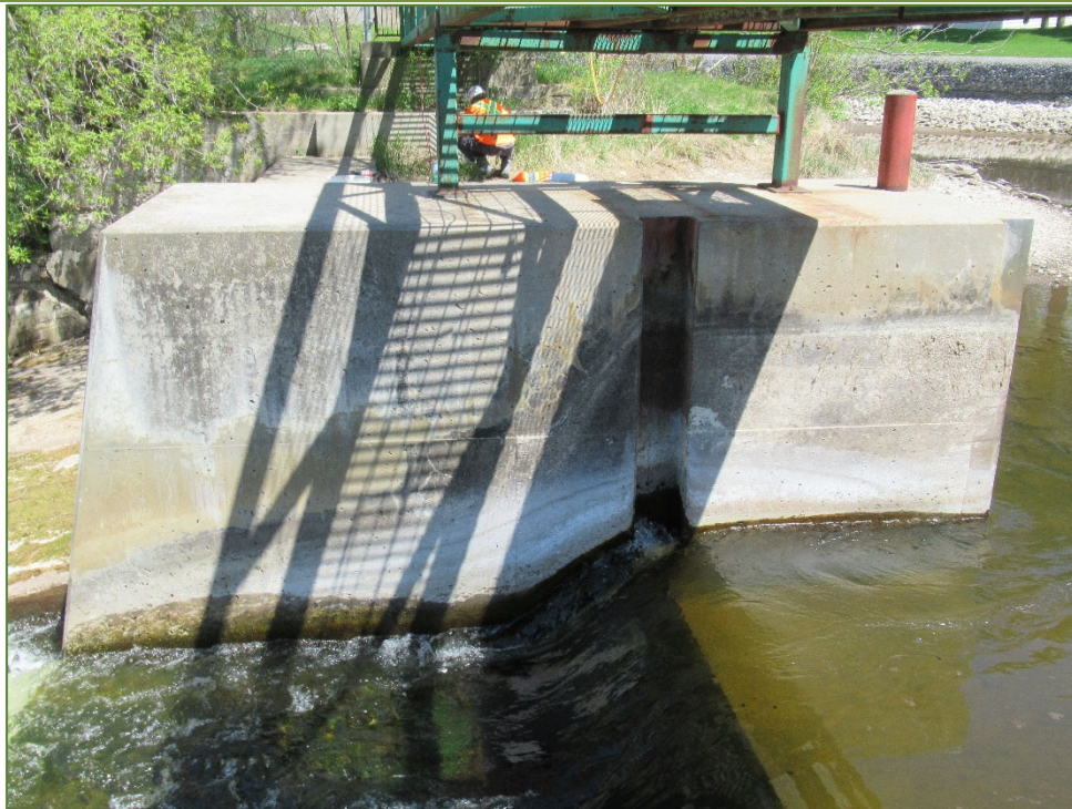
Photo P36 East Pier – West Face (fair to good condition – cracks, light scaling and wet stain)
