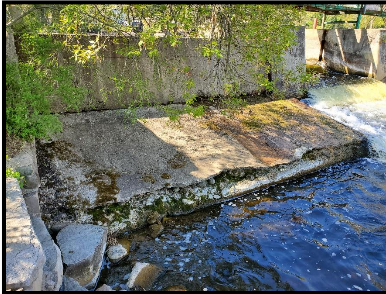
Photo 17 – East Concrete Apron, Severe Spalling and Undermining (Typ.)
