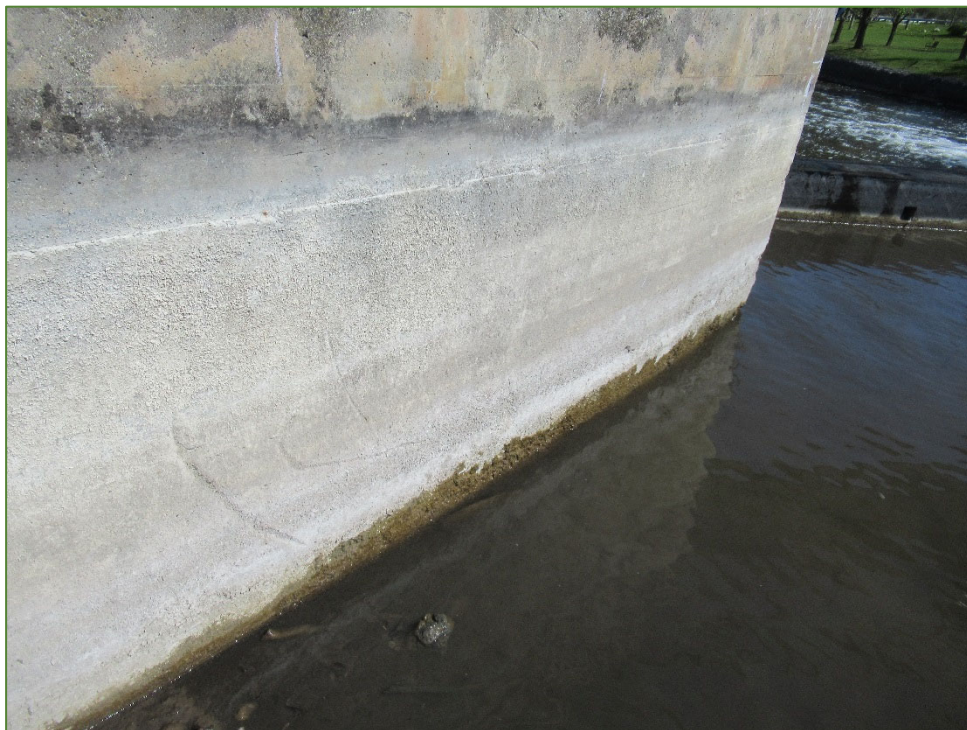
Photo P10 West Abutment and Retaining Wall (light scaling) note undermining
