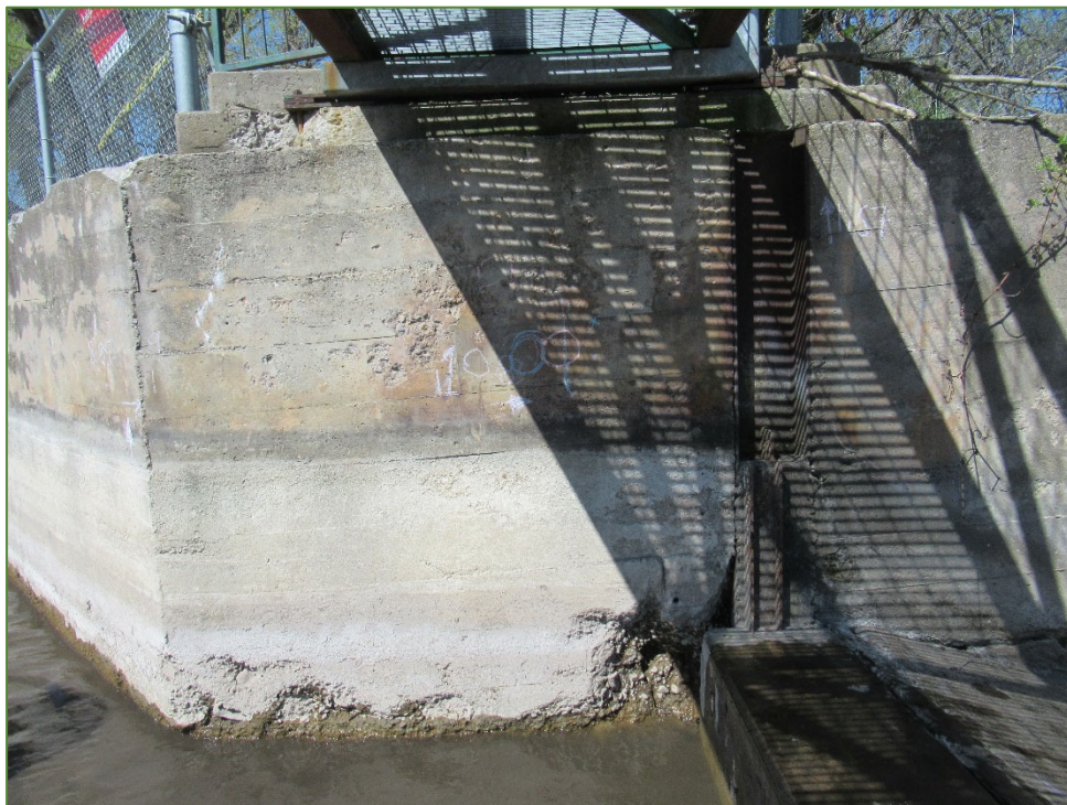
Photo P12 West Abutment and Retaining Wall (cracks, spall, light to severe scaling and staining) note undermining
