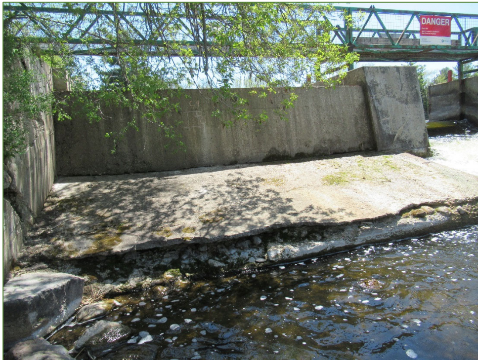
Photo P16 East Weir and Apron Slab, North Elevation (fair to poor condition – cracks, spall, delamination, honeycombing and light to medium scaling)
