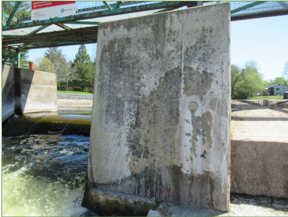
Photo P45 West Pier – North Face (fair to good condition – cracks, light scaling and wet stain)
