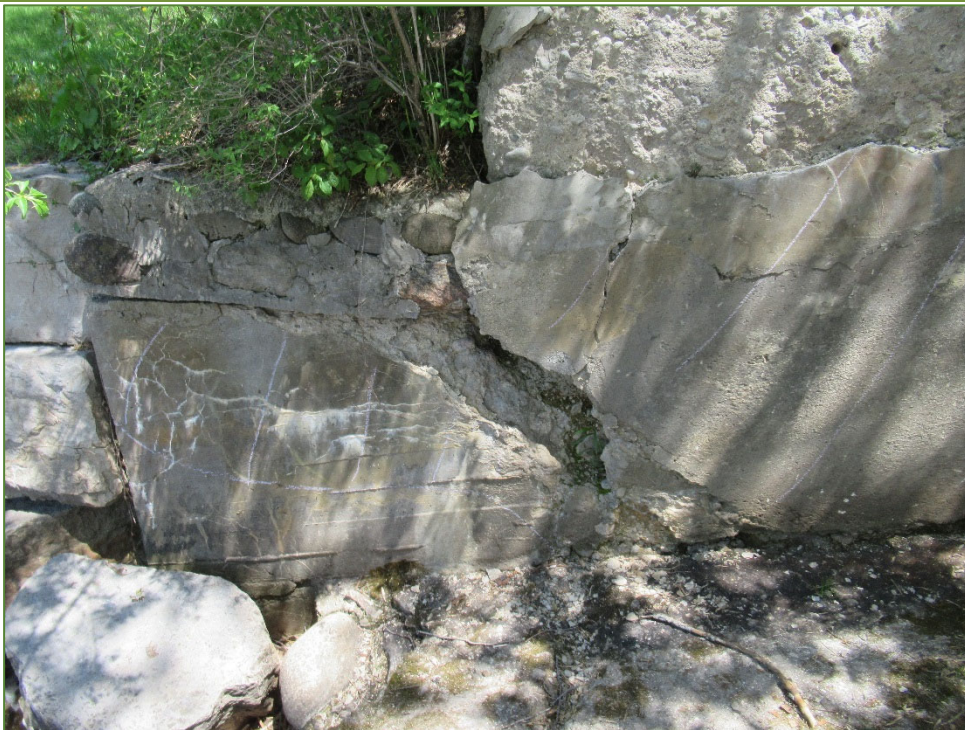
Photo P6 East Abutment and Retaining Wall (cracks, spall, delamination and light to severe scaling)
