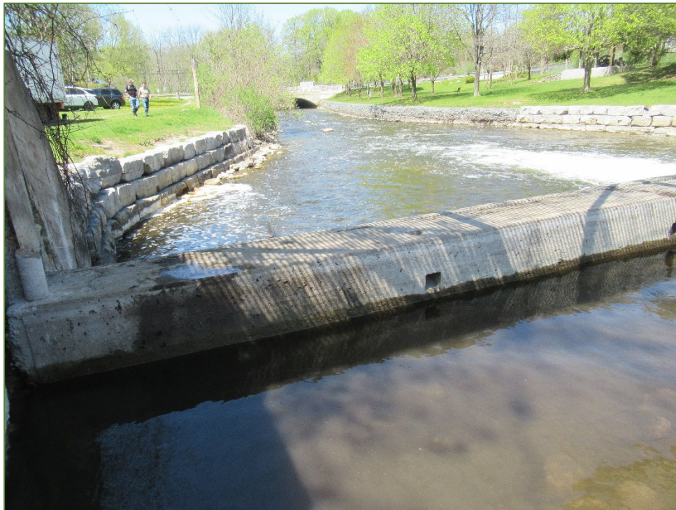
Photo P32 West Weir – South Elevation (spall and light scaling)
