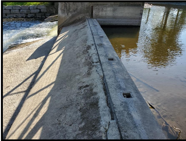
Photo 7 – West Overflow Weir, Wide Crack along Weir
