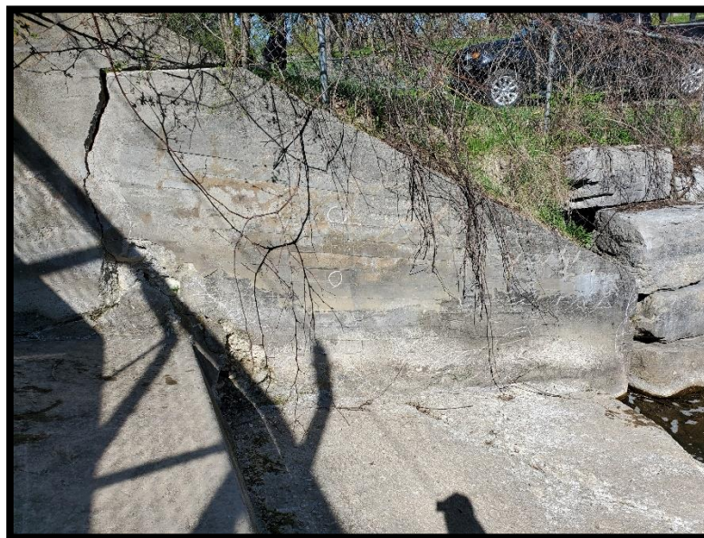
Photo 6 – Downstream Retaining Wall at West Abutment, Wide Vertical Crack and Spalling at Weir
