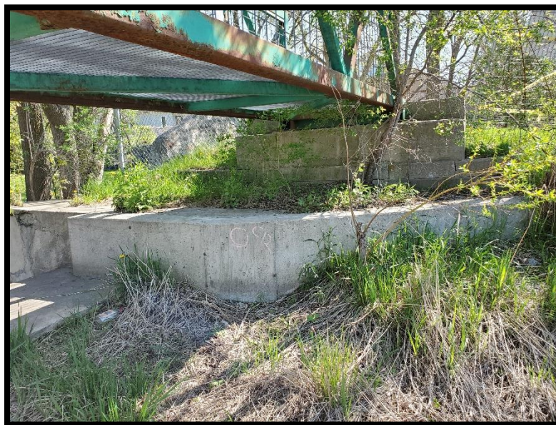
Photo 16 – East Abutment and Upstream Retaining Wall
