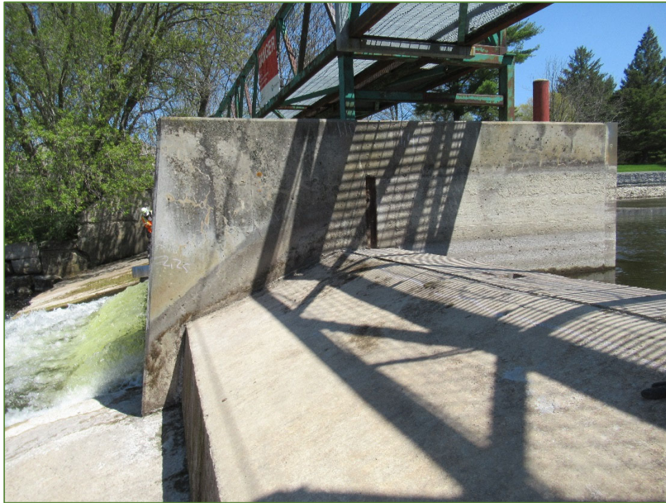
Photo P43 West Pier – West Face (fair to good condition – cracks, light scaling and wet stain)
