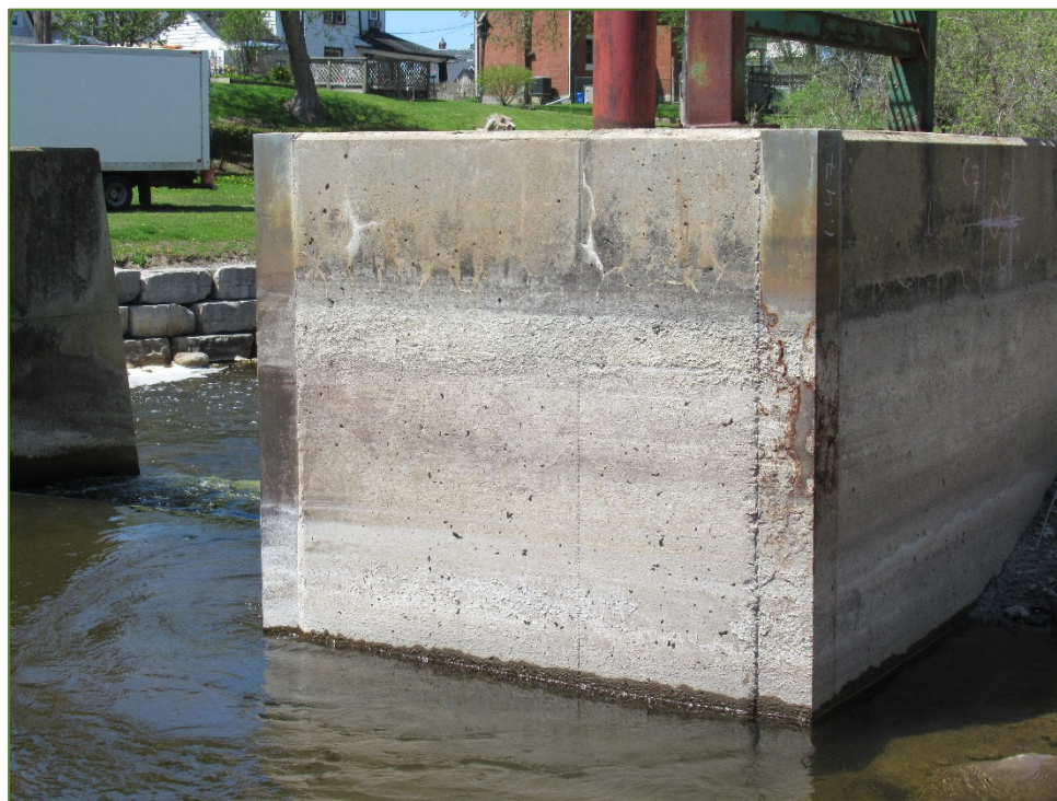
Photo P38 East Pier – South Face (fair to good condition - cracks, light scaling and wet stain )
