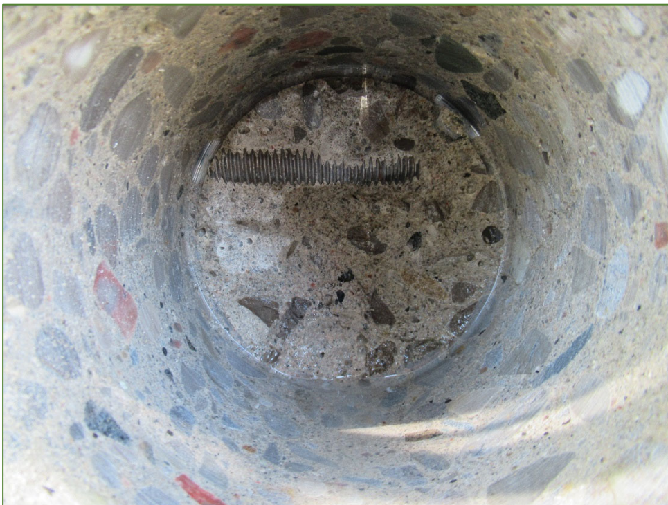
Photo P52 Typical Condition of Inside Core – C12
