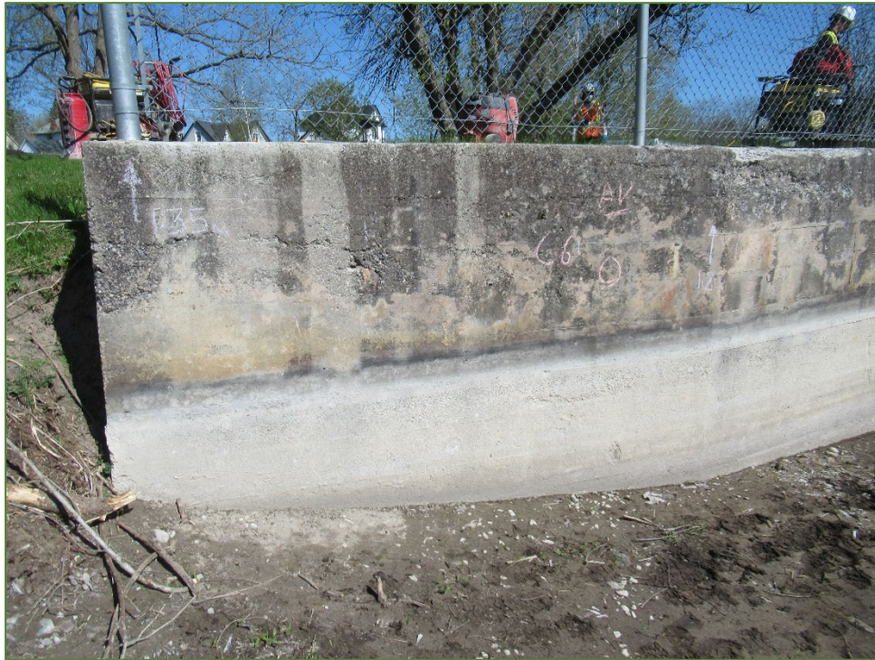
Photo P9 West Abutment and Retaining Wall (cracks, spall and light to medium scaling)
