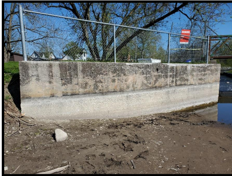
Photo 3 – Upstream West Retaining Wall, Spalling at Top Edge
