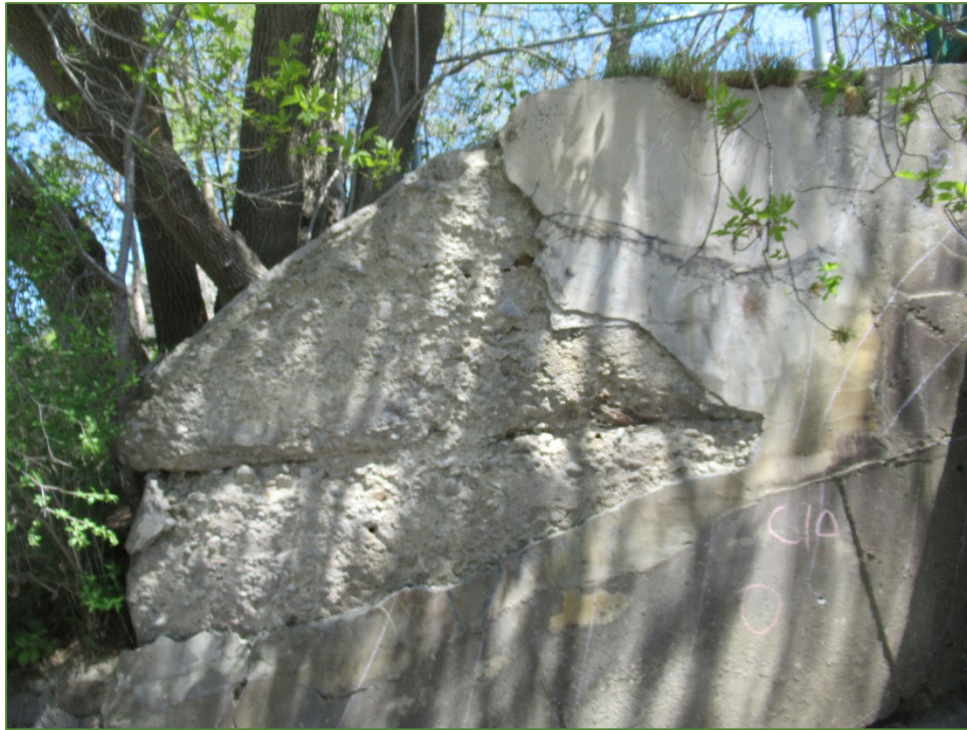
Photo P7 East Abutment and Retaining Wall (cracks, delamination and severe scaling)
