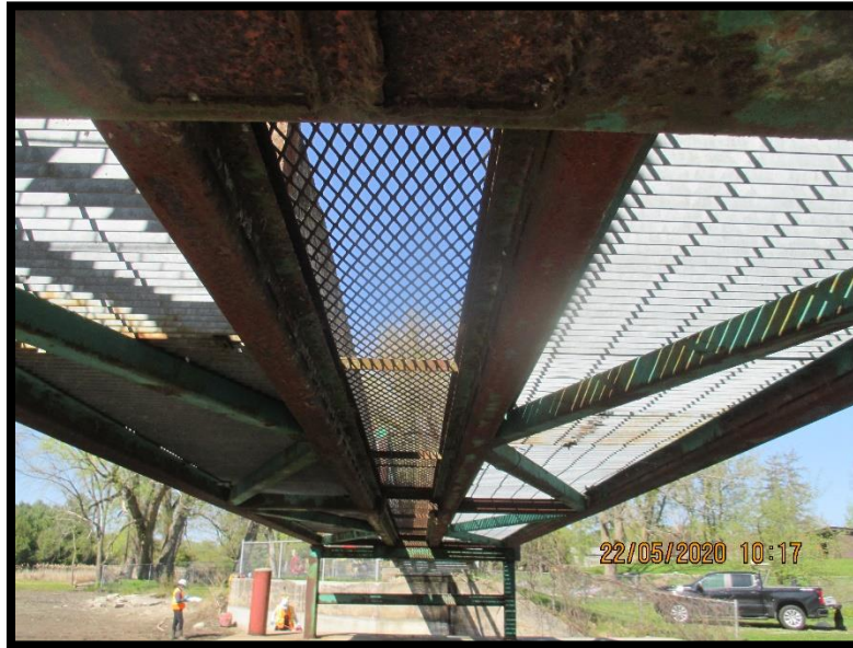
Photo 13 – Underside of Pedestrian Bridge over Operational Span, Failing Protective Coating and Moderate Corrosion of Longitudinal HSS (Typ.)
