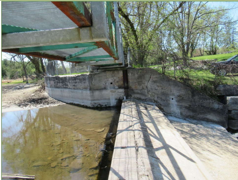
Photo P8 West Abutment and Retaining Wall (fair condition – cracks, spall, delamination, light to medium scaling and staining) note undermining, and alkali aggregate reaction on the surface
