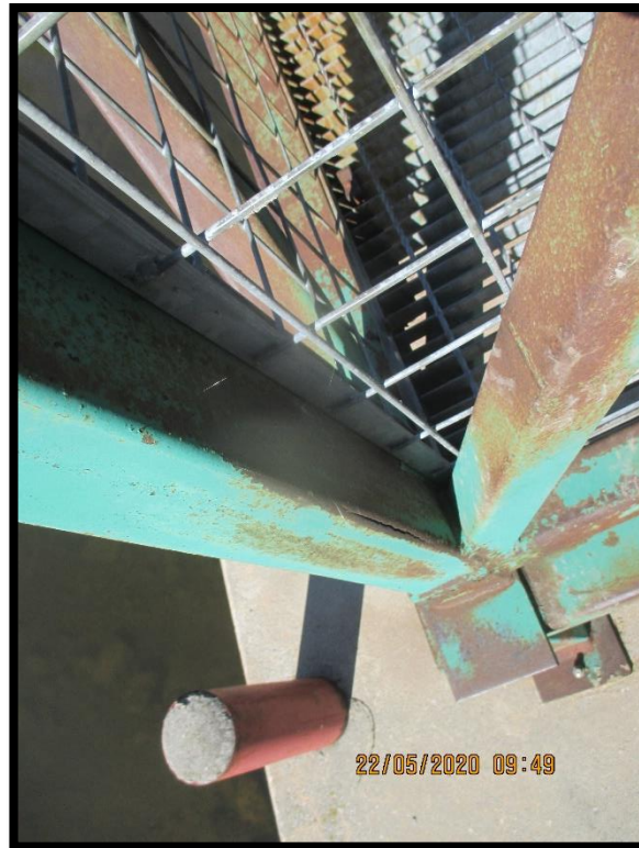
Photo 25 – Vertical HSS at Operational Span, Wide Cracks in Steel (3)
