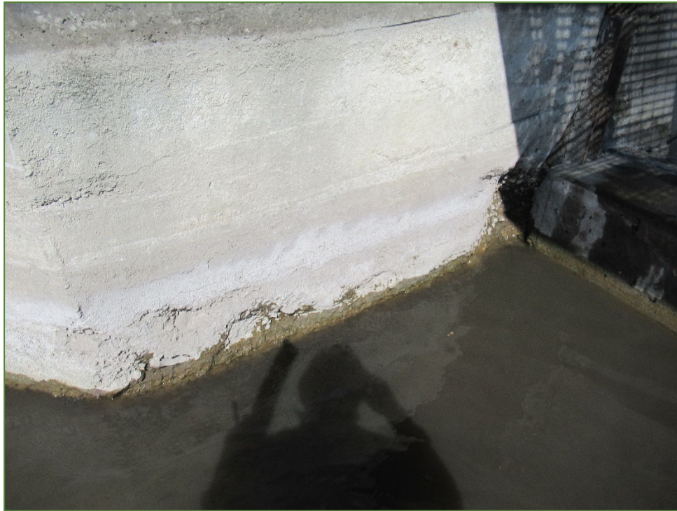
Photo P11 West Abutment and Retaining Wall (severe scaling) note undermining
