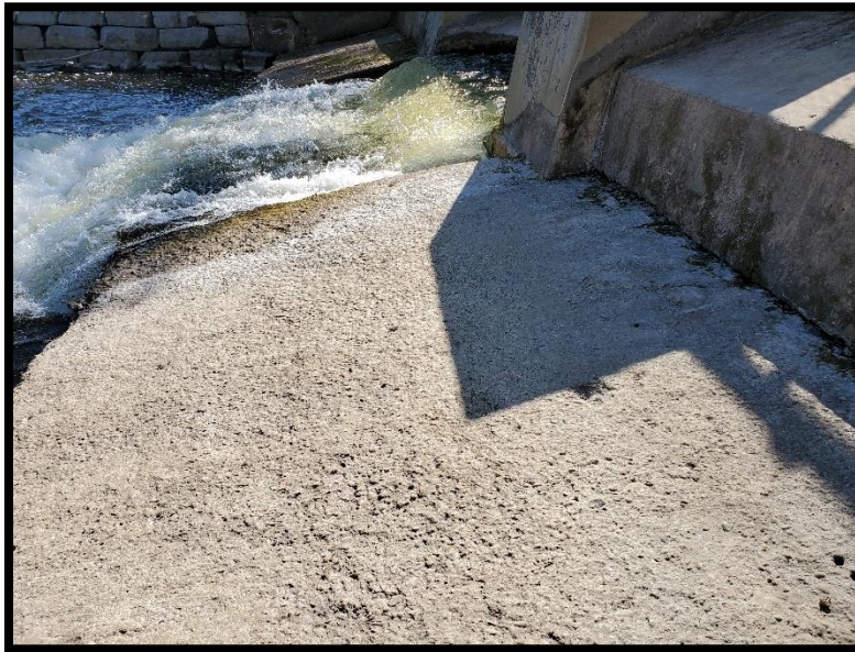
Photo 8 – West Overflow Weir Concrete Apron, Severe Scaling (Typ.)
