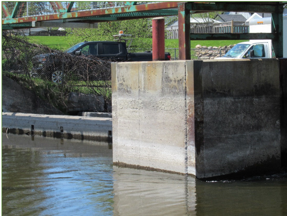
Photo P44 West Pier – South Face (fair to good condition – cracks, light scaling and wet stain)
