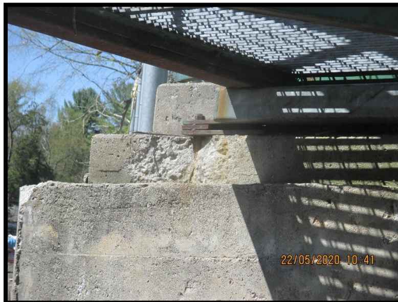
Photo 5 – West Abutment, Spalling Under Southwest Bearing
