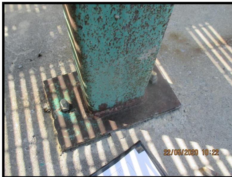
Photo 12 – Bearing Anchorage of HSS Support (Typ.)
