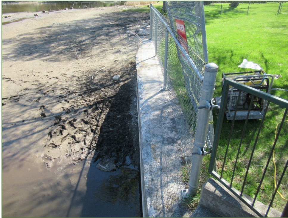
Photo P15 West Abutment and Retaining Wall – Top Face (spall and light scaling)
