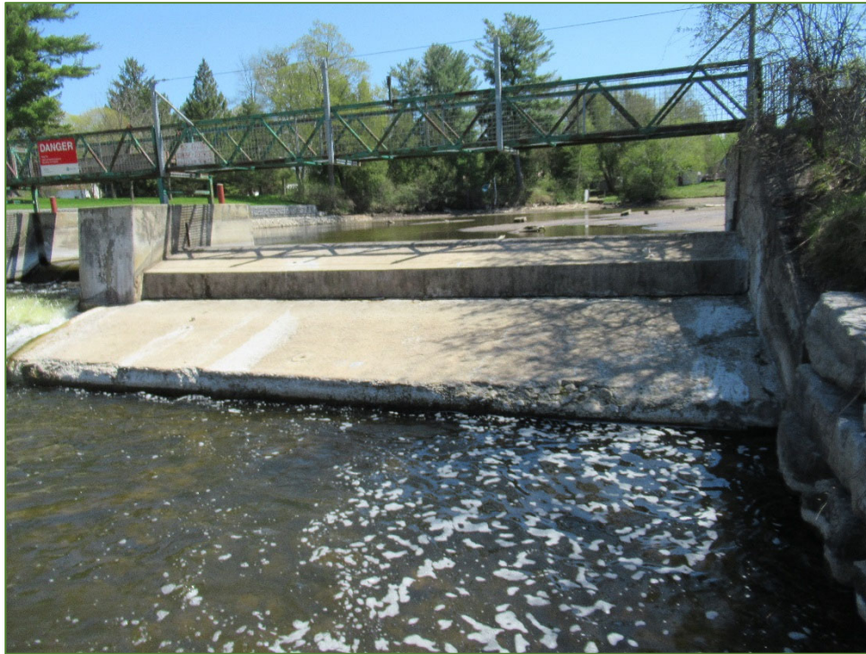
Photo P27 West Weir and Apron Slab – North Elevation (fair to poor condition – spall and medium scaling)
