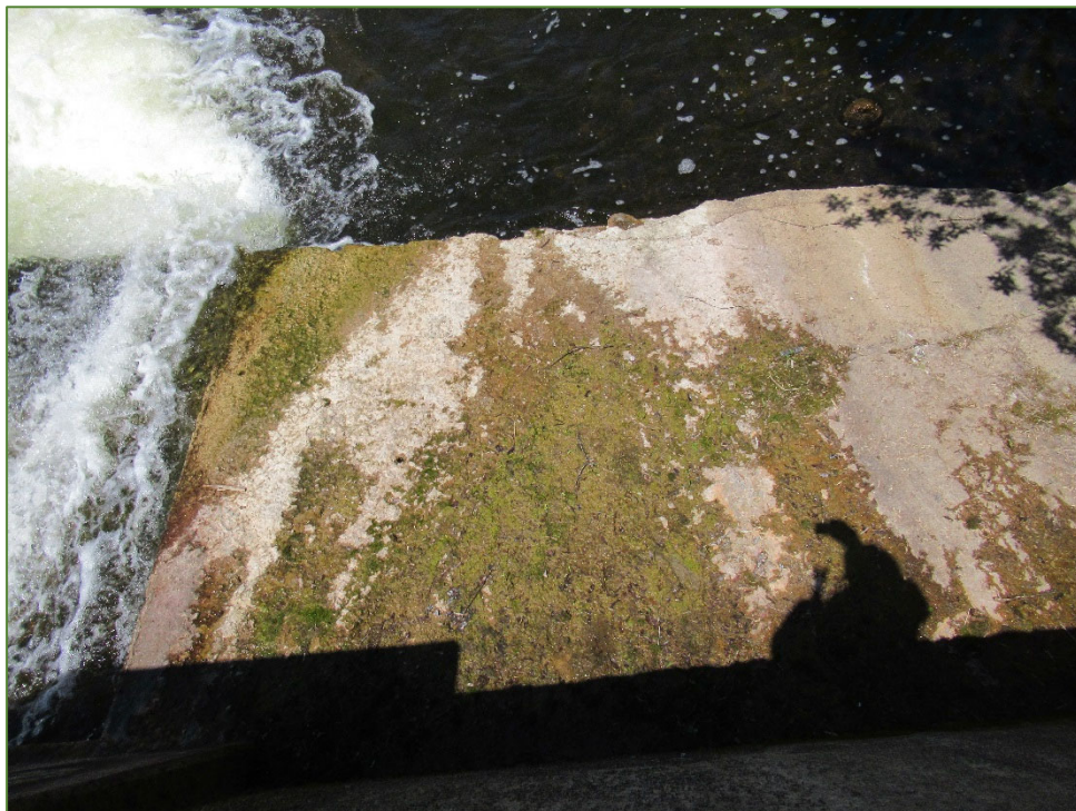
Photo P20 East Apron Slab Plan (cracks, spall and light scaling and staining)
