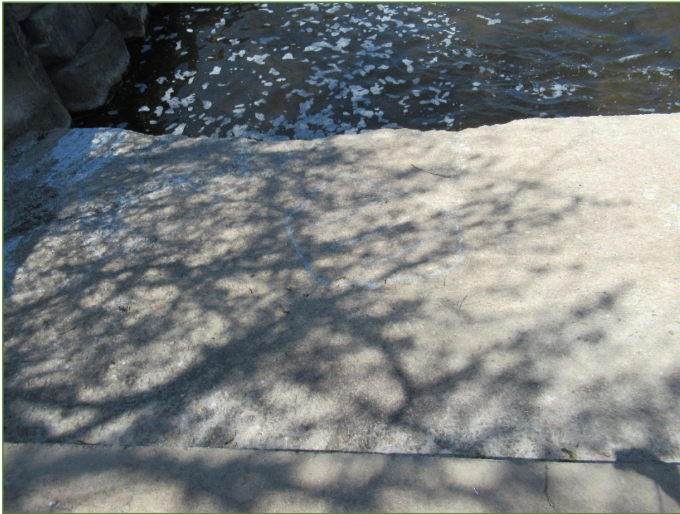
Photo P25 West Apron Slab Plan (spall, delamination and medium scaling)
