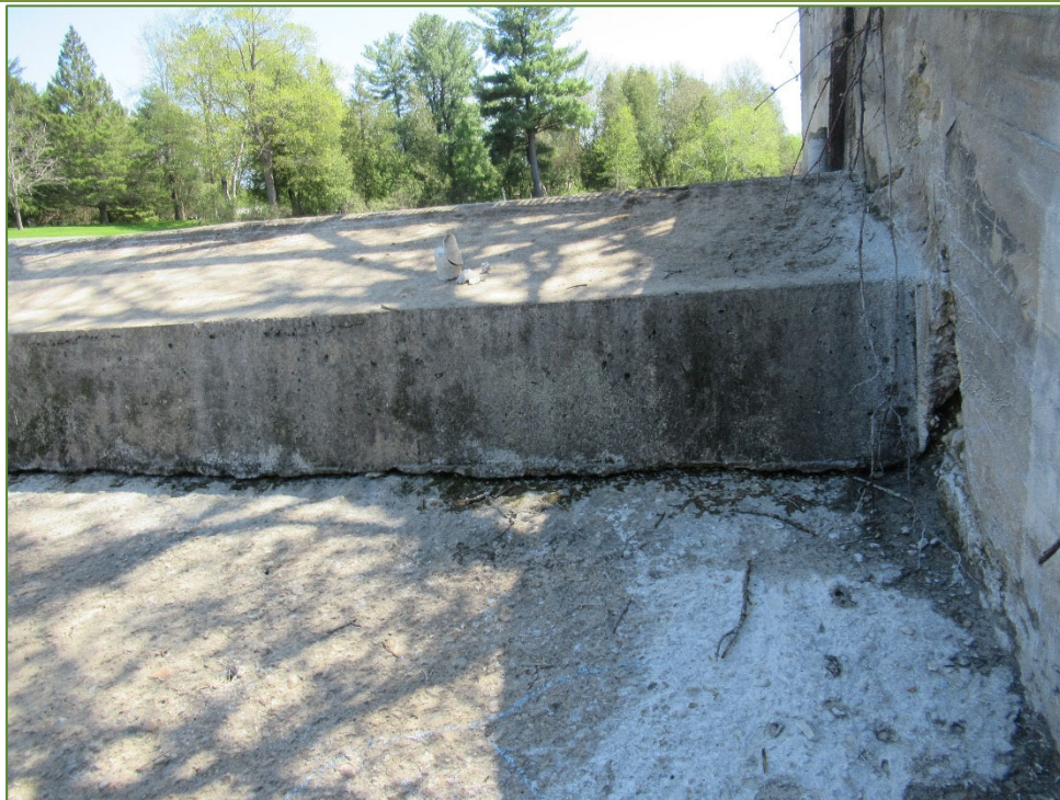
Photo P28 West Weir and Apron Slab – North Elevation (spall, delamination and medium scaling) note, undermining
