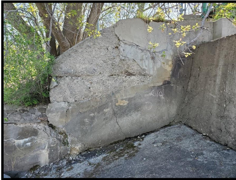
Photo 19 – Downstream East Retaining Wall, Severe Spalling, Disintegration, and Delamination with Wide Cracks (Typ.)
