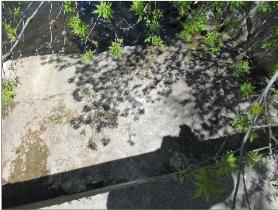
Photo P21 East Apron Slab Plan (cracks, spall and light scaling and staining)
