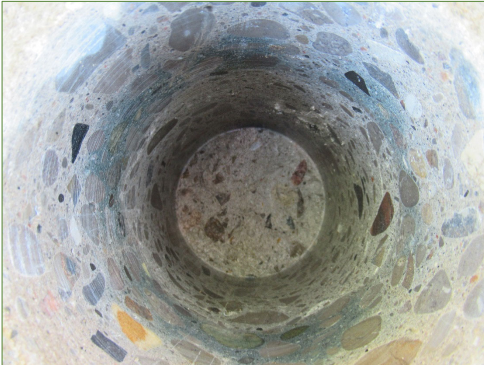
Photo P50 Typical Condition of Inside Core – C8
