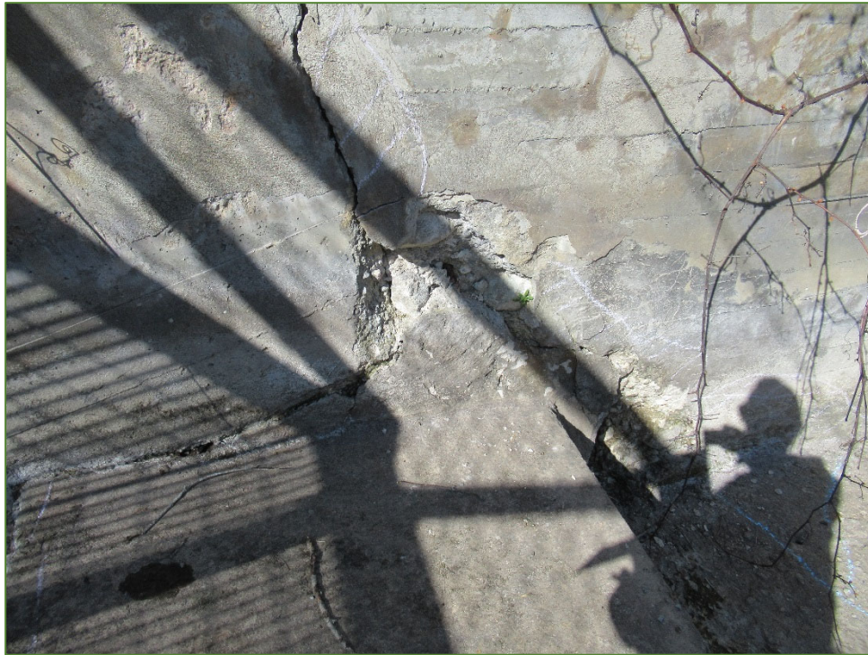
Photo P13 West Abutment and Retaining Wall (wide crack, spall and delamination)
