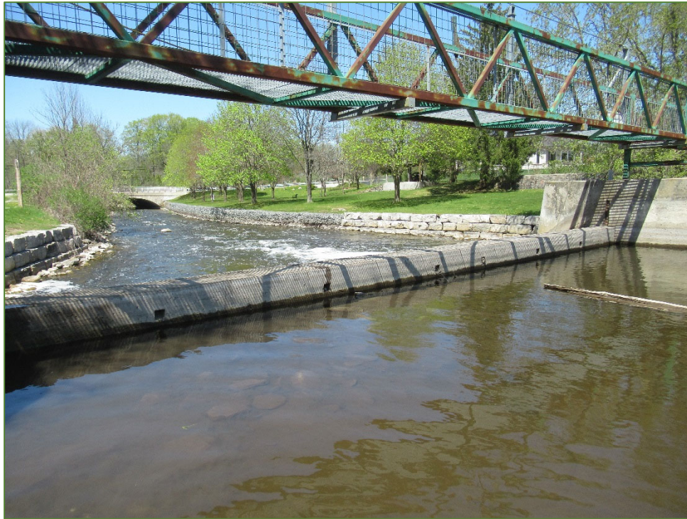
Photo P31 West Weir – South Elevation (good condition – spall and light scaling)
