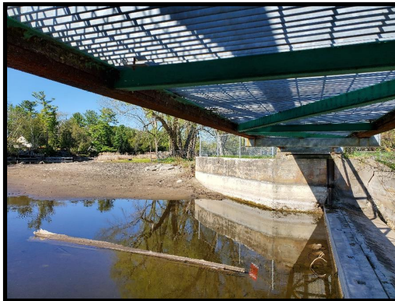
Photo 10 – Underside of West Span of Pedestrian Bridge, Failed Protective Coating and Moderate Corrosion of Longitudinal HSS (Typ.)
