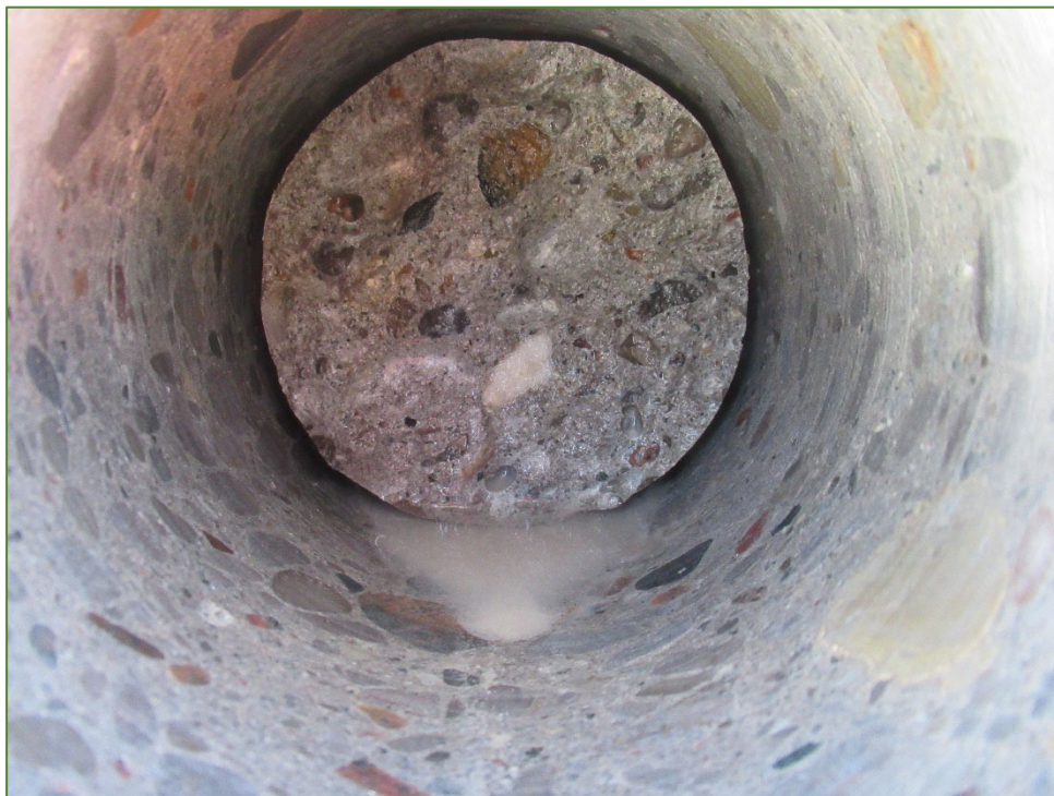
Photo P48 Typical Condition of Inside Core – C5
