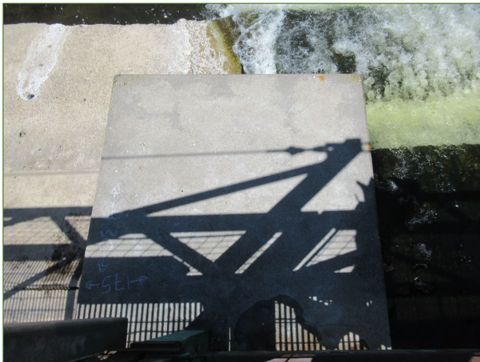
Photo P40 West Pier – Top Face (good condition - cracks and light scaling)
