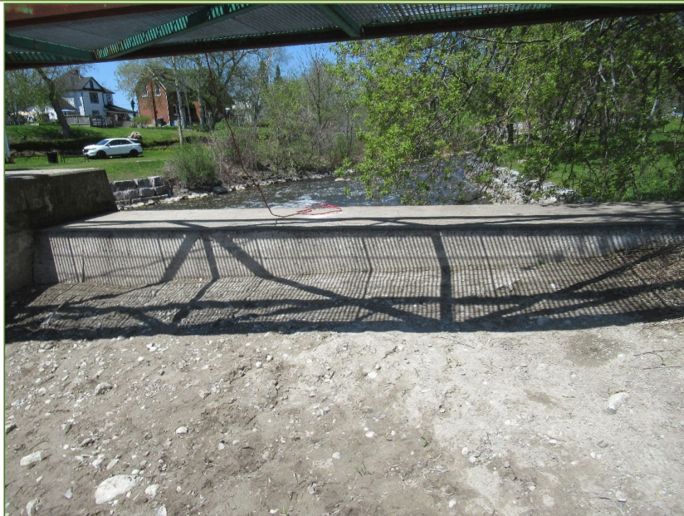
Photo P22 East Weir – South Elevation (good condition – light scaling)
