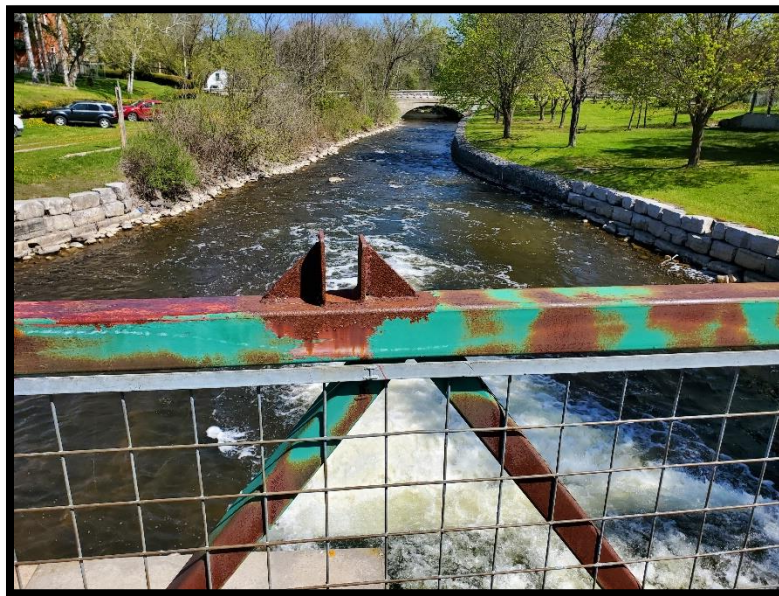
Photo 22 – Winch Anchorage on Truss HSS, Moderate Corrosion (Typ.)
