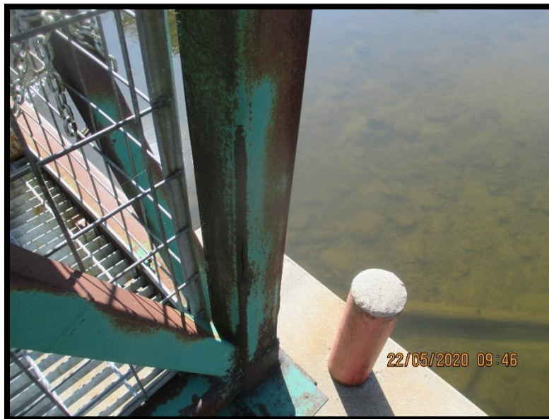
Photo 24 – Vertical HSS at Operational Span, Wide Cracks in Steel (2)
