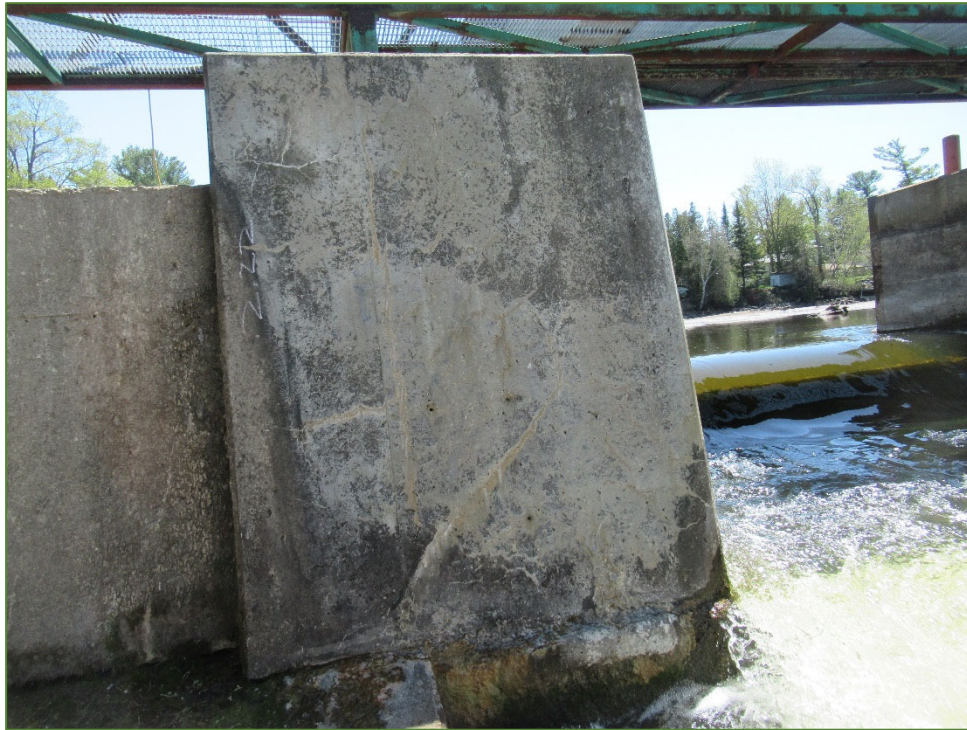
Photo P39 East Pier – North Face (fair condition - cracks, medium scaling and wet stain)
