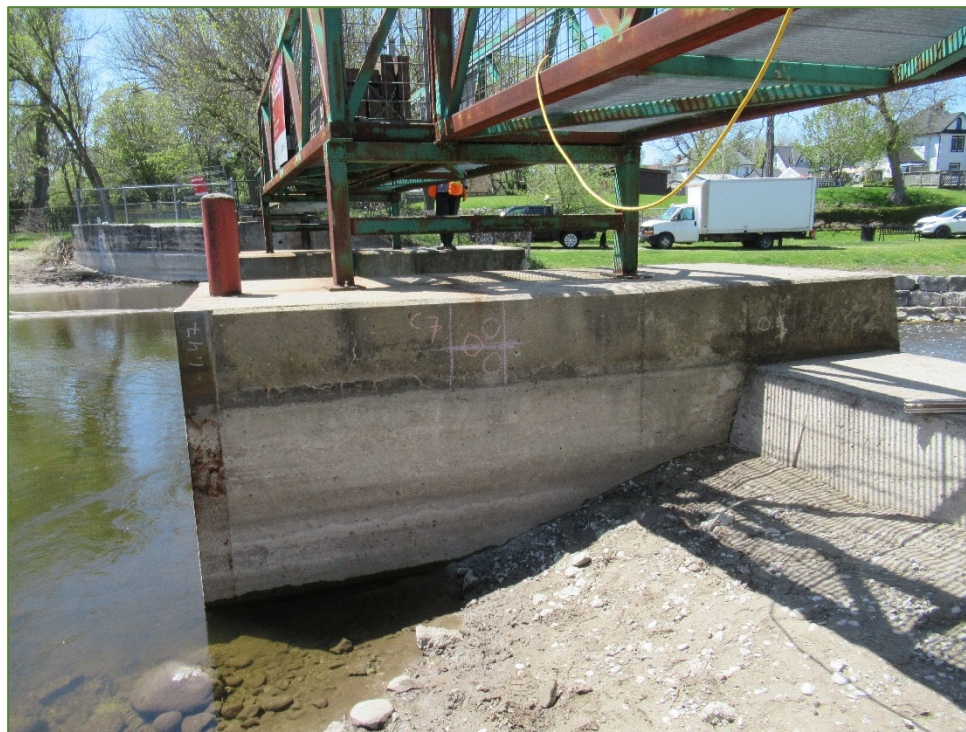
Photo P37 East Pier – East Face (fair to good condition – cracks, light scaling and wet stain)
