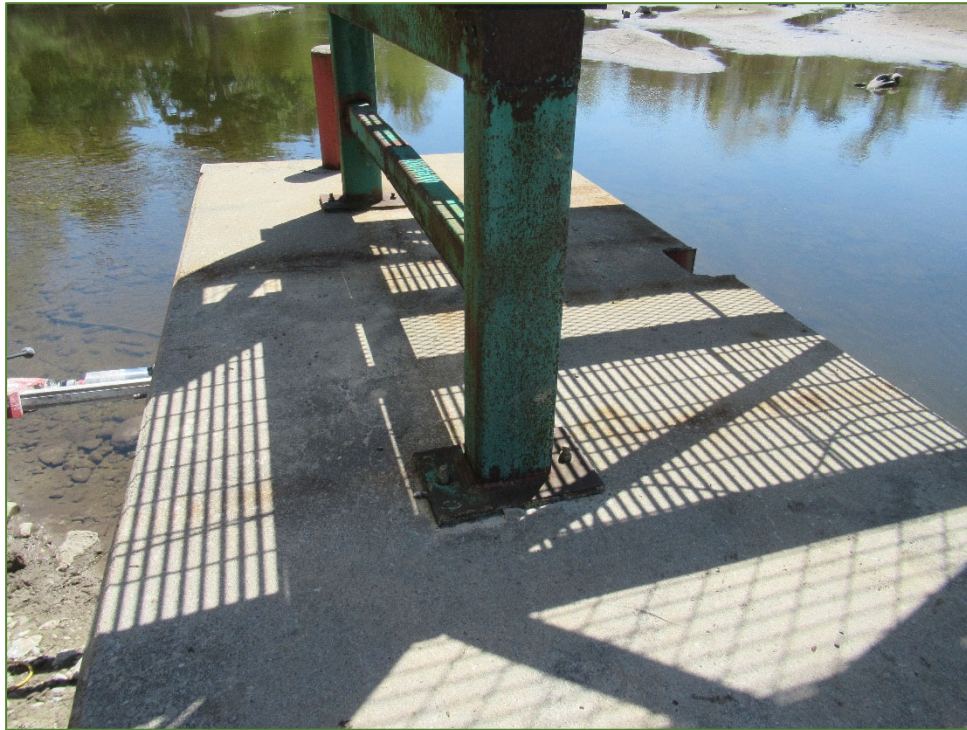
Photo P33 East Pier – Top Face (good condition – cracks and light scaling)
