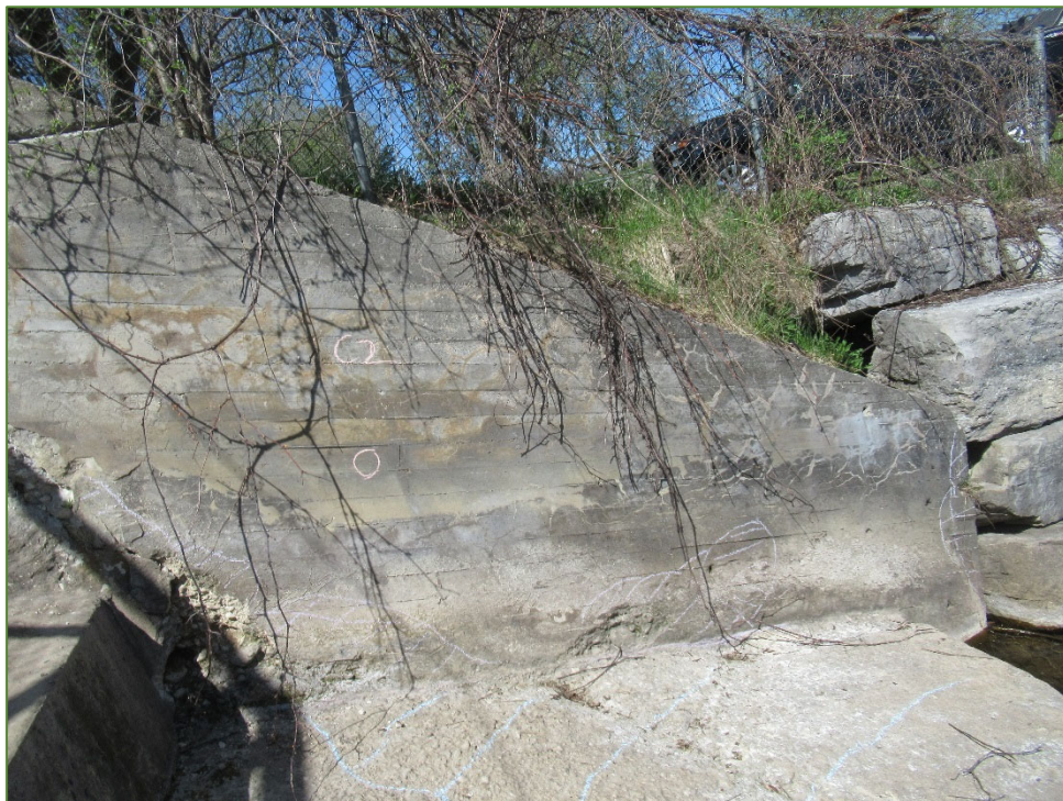
Photo P14 West Abutment and Retaining Wall (cracks, spall and delamination)
