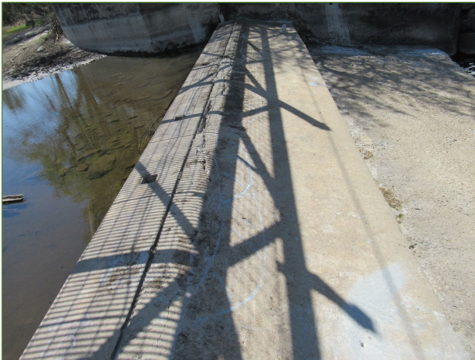
Photo P26 West Weir Plan (wide cracks, spall and delamination)
