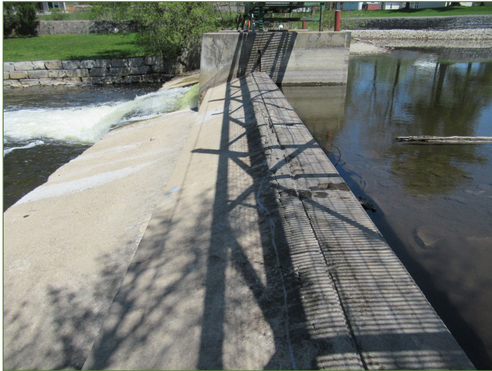
Photo P23 West Weir and Apron Slab Plan (poor condition – wide cracks, spall, delamination and light to medium scaling)
