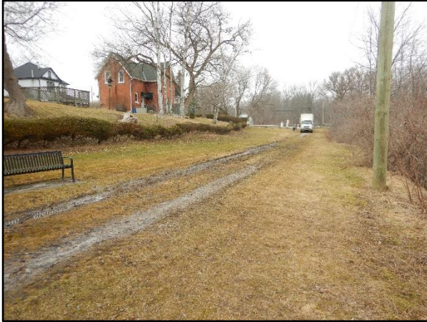
Photo 1 – Main Access Driveway, West Side of Dam
