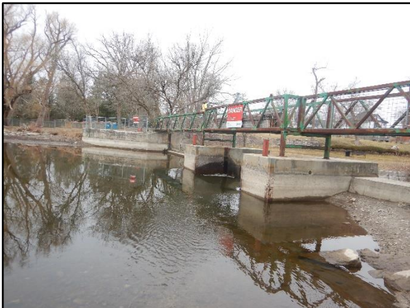
Photo 5 – Control Structure, Upstream
