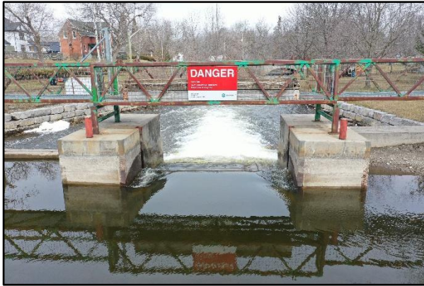
Photo 19 – Stoplog Sluiceway
