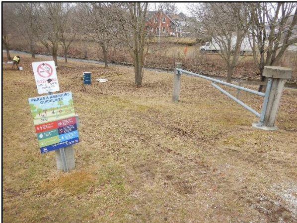
Photo 3 – Access gate, East Side of Dam
