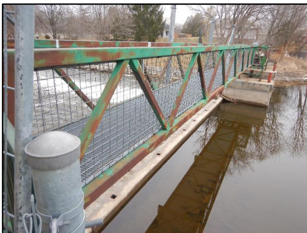
Photo 24 – Typical Truss Bridge Railing
