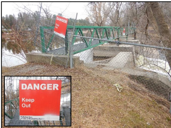
Photo 26 – Fencing and Sign on Right Side
