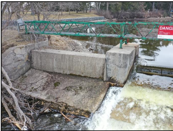
Photo 11 – East Concrete Weir
