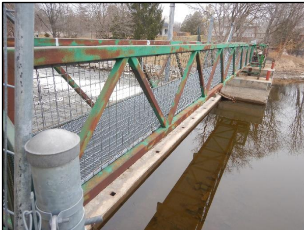
Photo 24 – Typical Truss Bridge Railing
