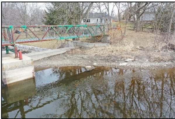
Photo 21 – East Concrete Weir
