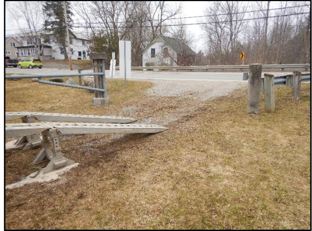
Photo 2 – Access Gate, West Side of Dam
