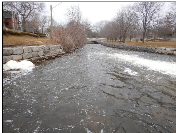
Photo 28 – Tailrace Channel and Retaining Walls
