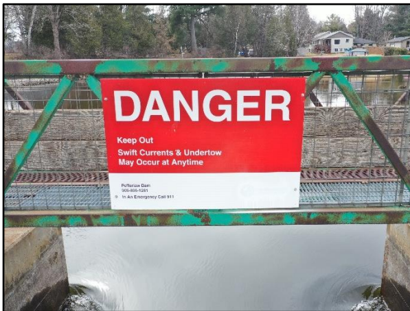
Photo 29 – Downstream Facing Public Safety Sign
