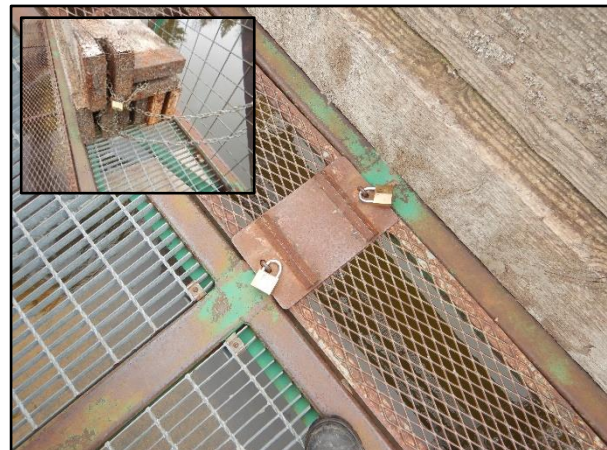
Photo 27 – Typical Stoplog and Gain Cover Locks
