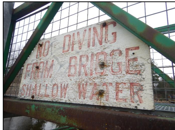
Photo 30 - Downstream Facing Public Safety Sign
