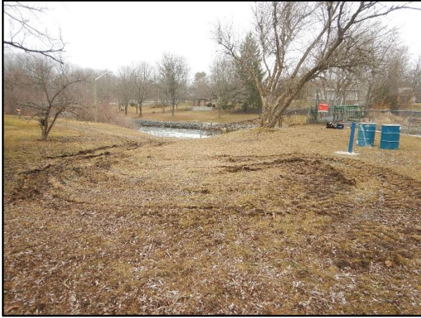
Photo 7 – West Earth Embankment
