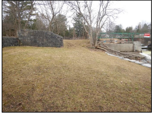
Photo 8 – East Earth Embankment
