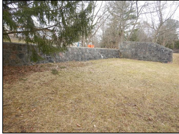
Photo 14 – Former Mill Structure
