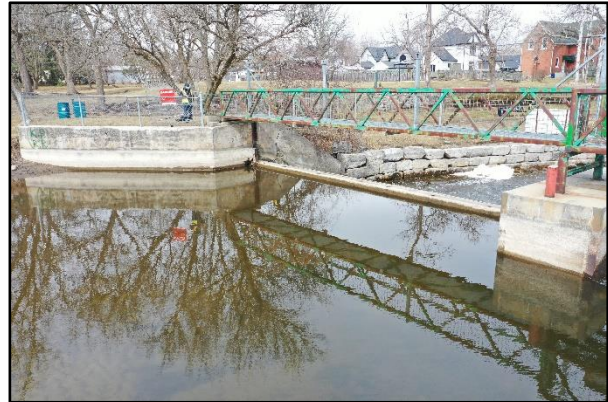
Photo 20 – Concrete Weir with Flashboards
