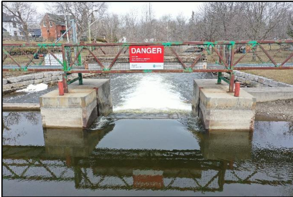
Photo 19 – Stoplog Sluiceway
