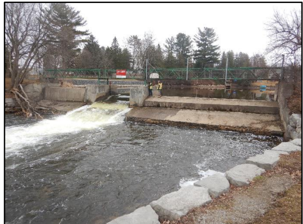
Photo 6 – Control Structure, Downstream
