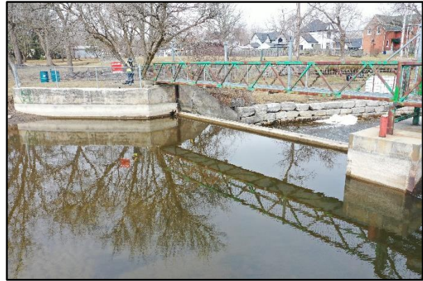
Photo 20 – Concrete Weir with Flashboards
