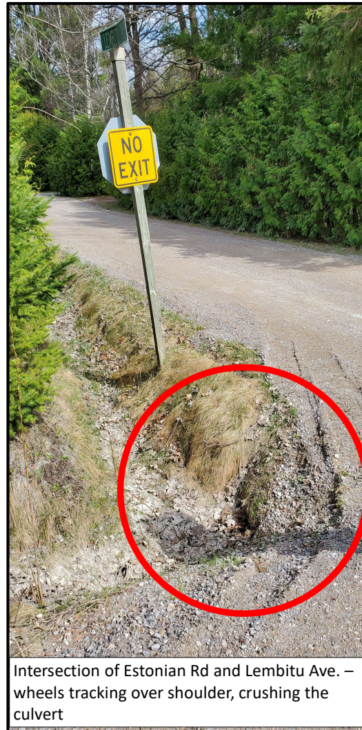
Intersection of Estonian Rd and Vambola Ave – wheels tracking over shoulder, crushing the culvert
