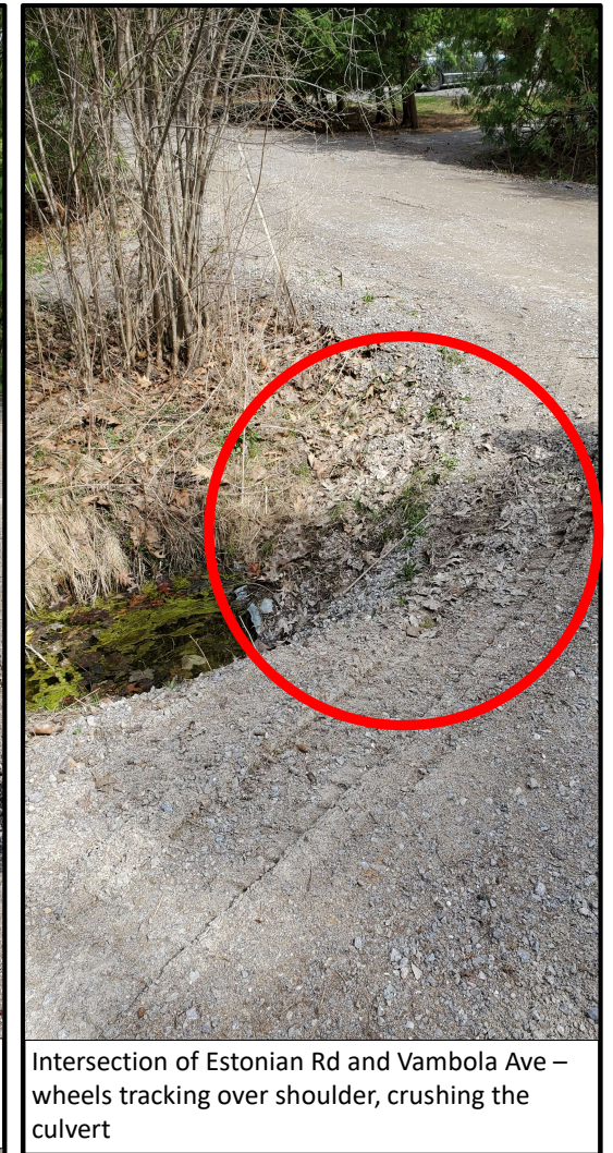
Intersection of Estonian Rd and Lembitu Ave. – wheels tracking over shoulder, crushing the culvert
