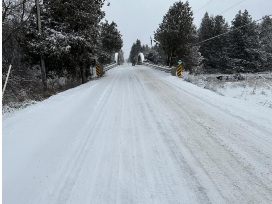
Plate 1 View of West Approach (Facing East)
