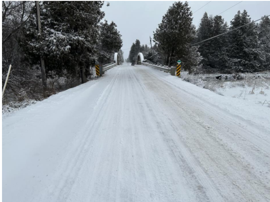
Plate 1 View of West Approach (Facing East)
