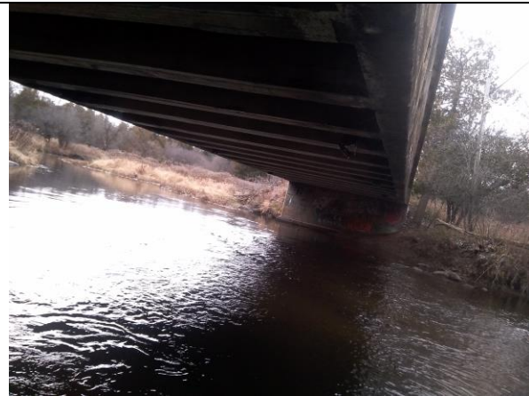
IMAGE 5 UNDERSIDE OF OLD SHILOH BRIDGE EAST
