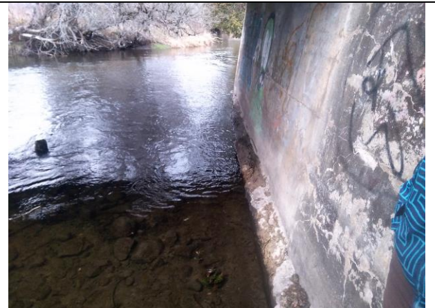
IMAGE 6 CONCRETE PILASTER OF OLD SHILOH BRIDGE EAST
