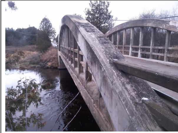
IMAGE 7 VIEW OF CONCRETE BOWSTRING ARCH OF OLD SHILOH BRIDGE EAST
