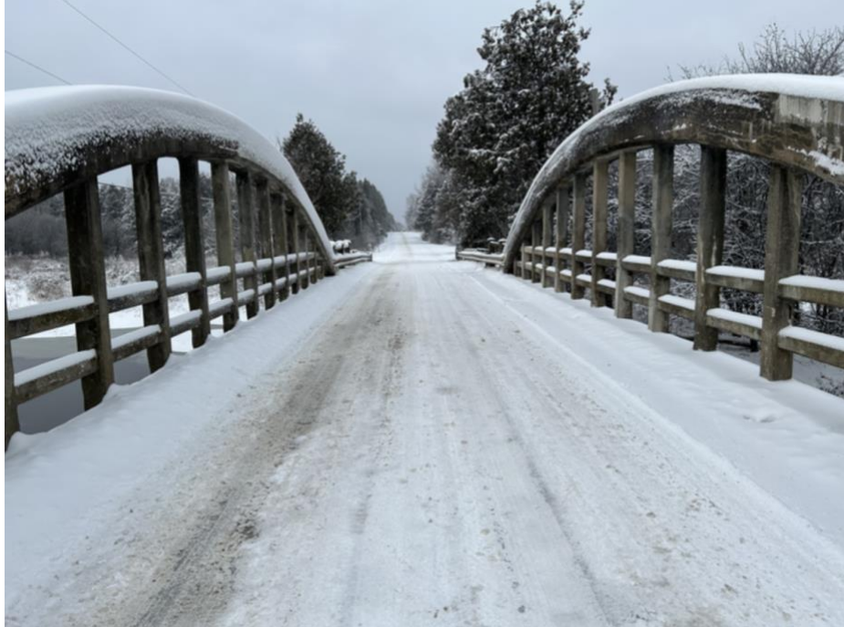
Plate 5 View of Deck (Facing West)
