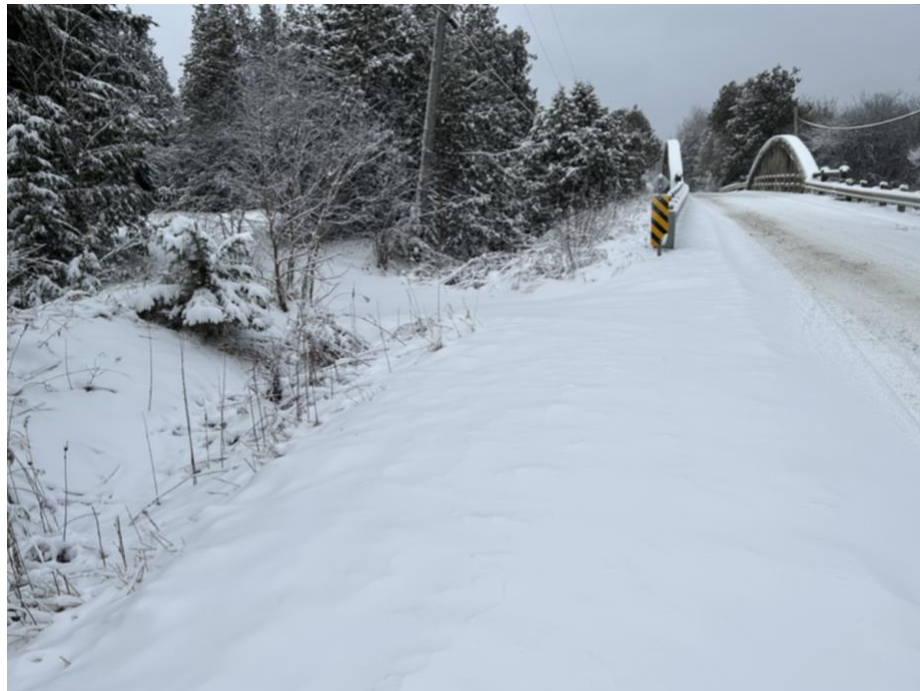
Plate 8 View of Western Approach (Facing East)
