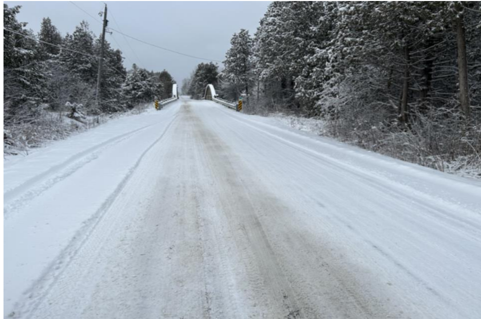
Plate 2 View of East Approach (Facing West)
