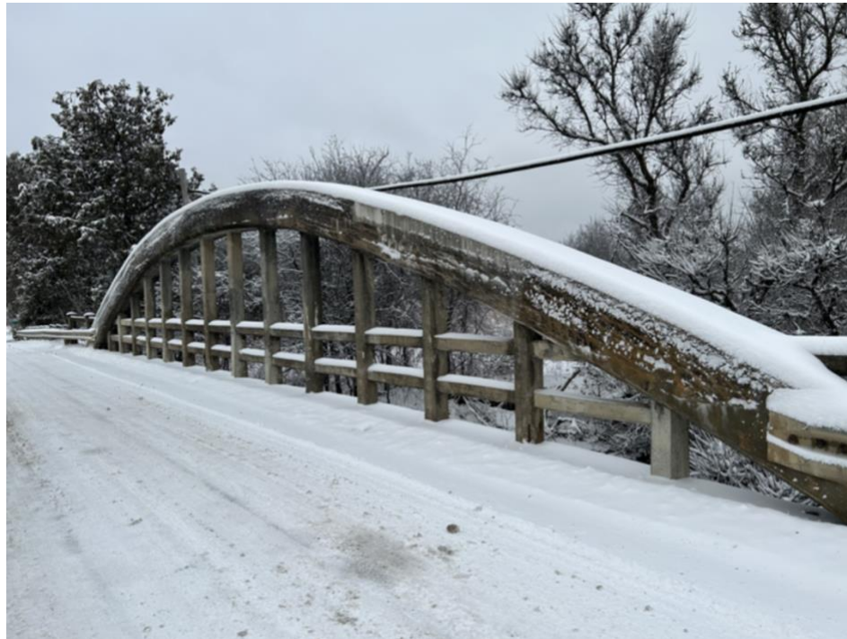
Plate 3 View of Deck (Facing Northwest)
