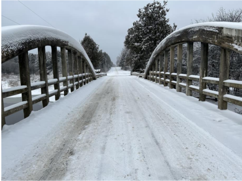
Plate 5 View of Deck (Facing West)
