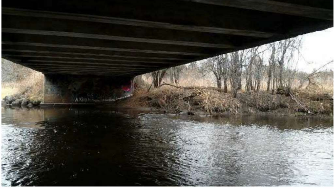
Photo 7. Facing west underneath bridge.
