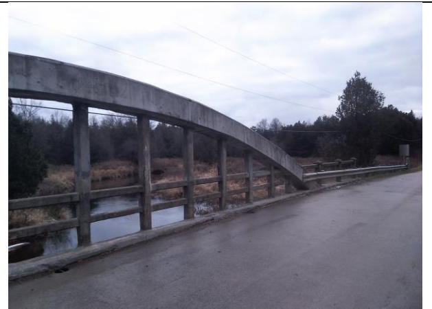
IMAGE 2 VIEW OF CONCRETE BOWSTRING ARCH OF OLD SHILOH BRIDGE EAST
