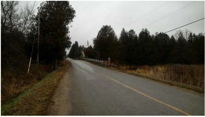
Photo 1. Facing east towards crossing.
