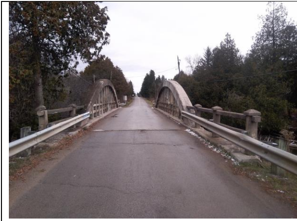
IMAGE 1 VIEW OF OLD SHILOH BRIDGE EAST
