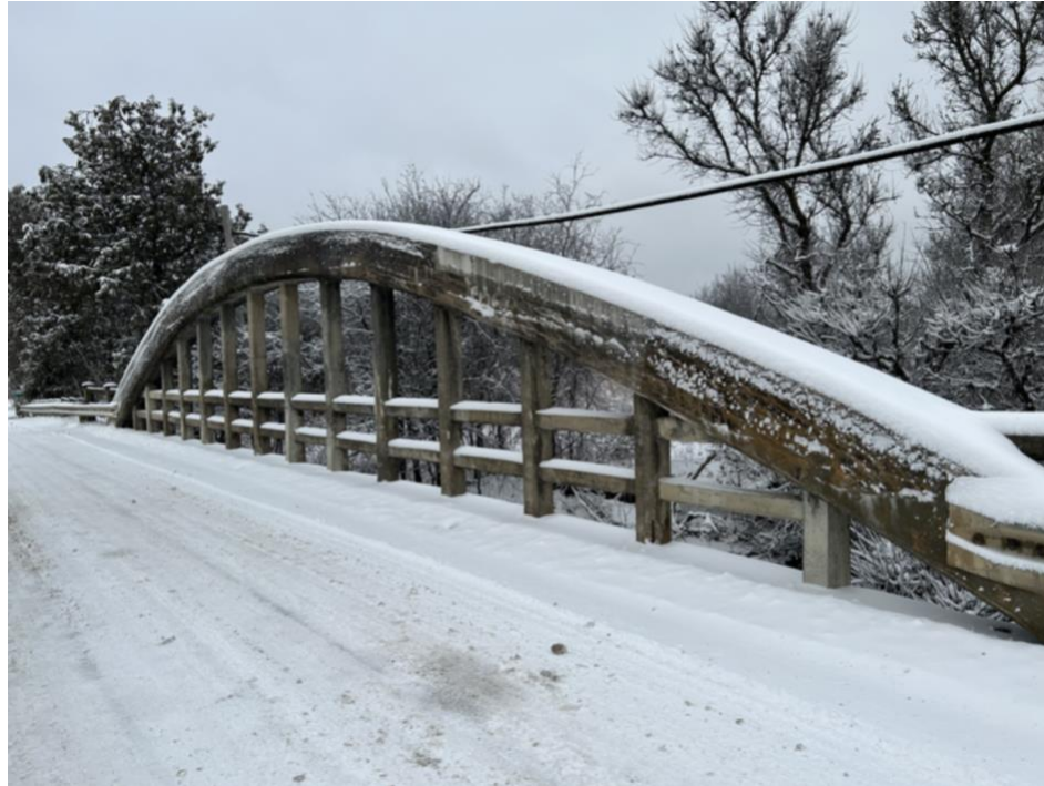
Plate 3 View of Deck (Facing Northwest)
