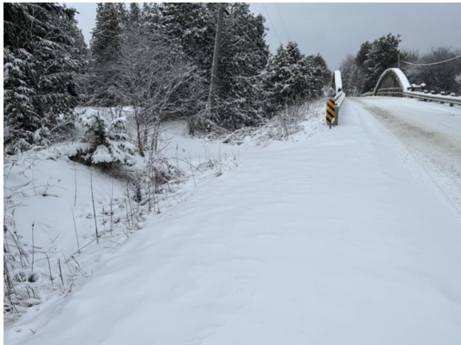
Plate 8 View of Western Approach (Facing East)
