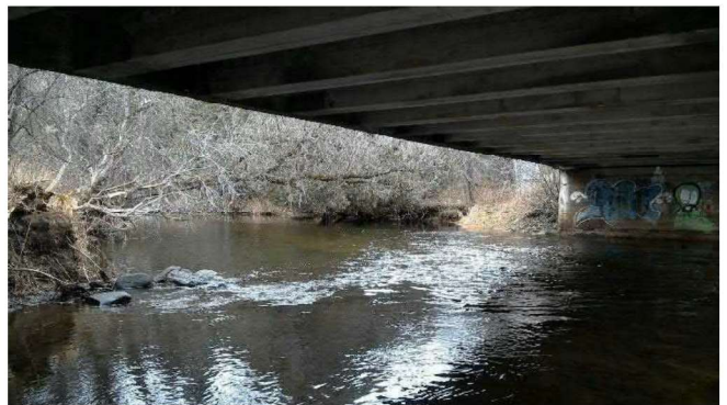
Photo 6. Facing northeast from underneath bridge.
