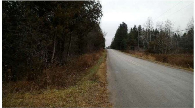
Photo 14. Facing east from east side of bridge.
