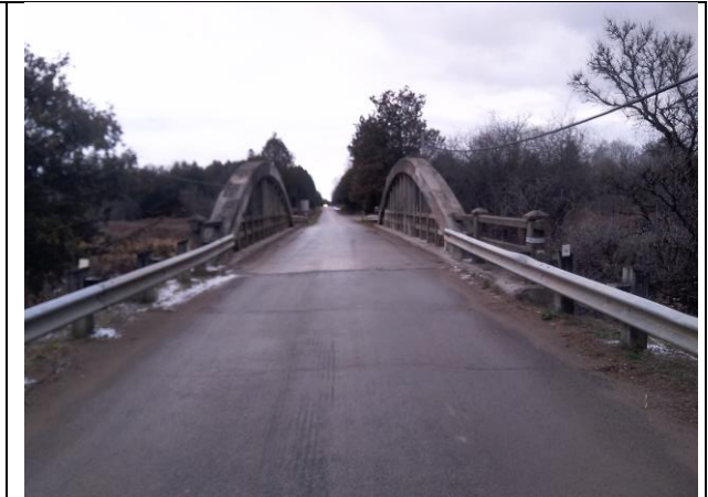
IMAGE 8 OVERVIEW OF OLD SHILOH BRIDGE EAST
