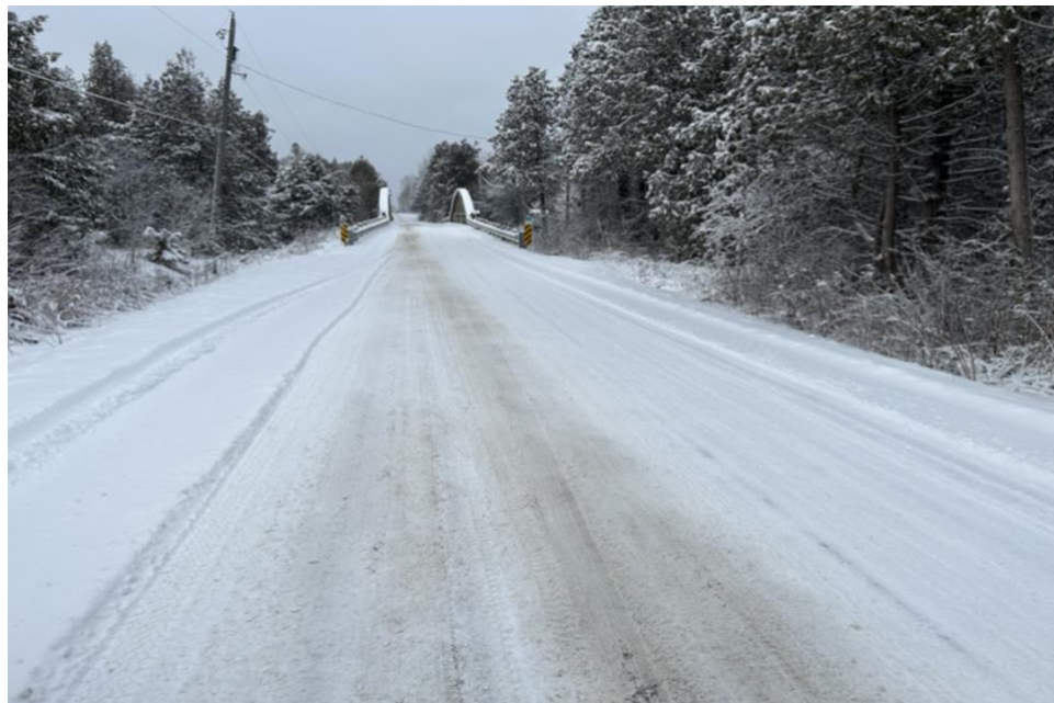
Plate 2 View of East Approach (Facing West)
