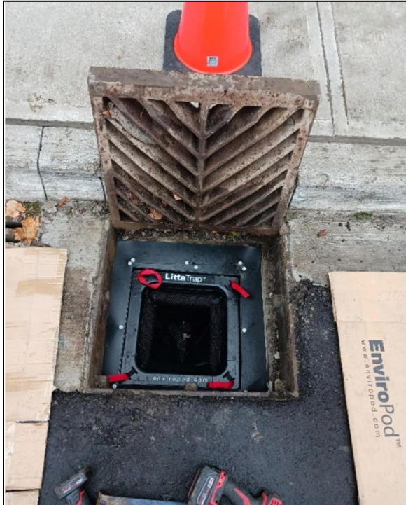
Figure 2: Catch-basin filter installed in November 2023 on Lake Drive in Jackson's Point
