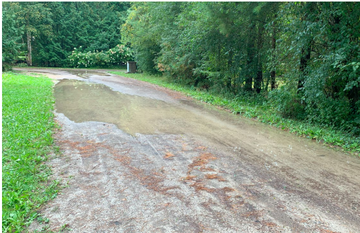
Figure 3: Poorly drained segment of Udora gravel road
