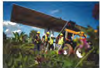
Solar panel installation in southwestern Ontario
