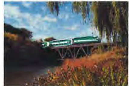
GO transit on the Milton rail corridor
