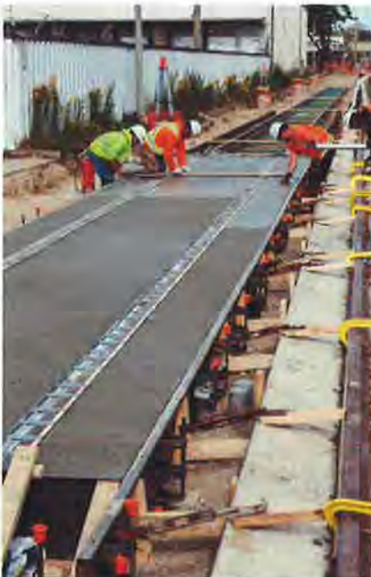
Light rail transit construction, Region of Waterloo
