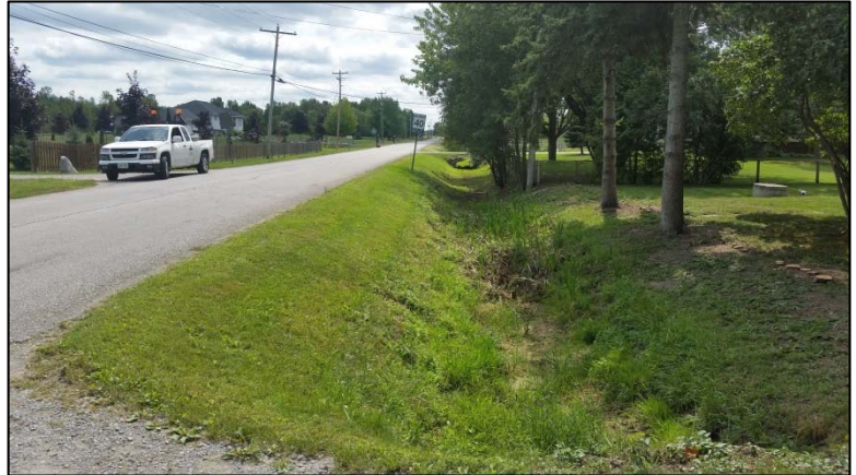
Figure 1.1: Standing water in roadside ditch.
