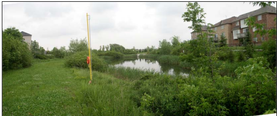
Figure 8.31: Grass Cutting along Walkways, Access and Inspection Areas. Grass has been left long adjacent to the permanent pool to deter geese.
