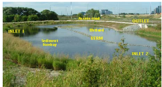
Figure 6.12: Typical Wet Pond.
