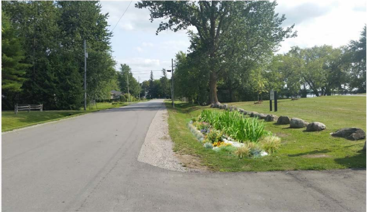
Figure 8.23: An opportunity for the implementation of a bioretention unit was identified on Ways Bay Drive. This location is adjacent to Claredon Beach Park, a community focal point of Keswick. Bioswales and bioretention areas can be incorporated into the park planting plans.
