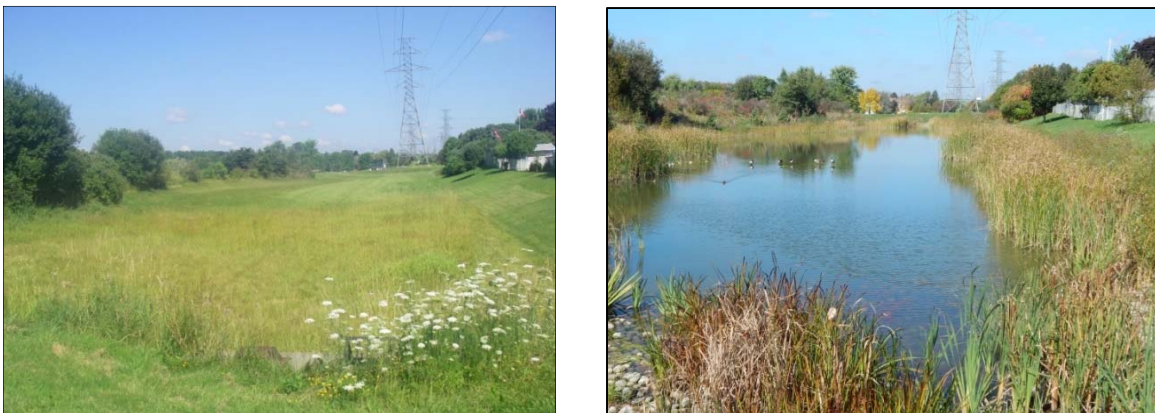
Figure 8.25: Retrofit of a Dry Stormwater Detention Facility (left) to a Wet SWM Facility (right).
