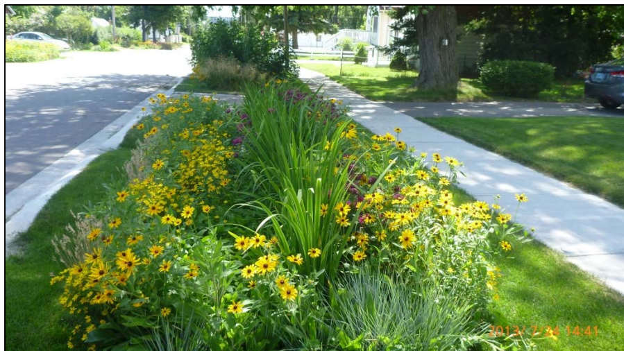
Bioretention systems and bioswales are part of the suite of best management practices (BMPs), known as LID, that promote infiltration/groundwater Figure 3.1: Bioretention at Lakeview in Mississauga.
