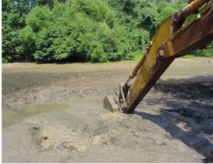
Figure 8.32: Sediment Dredging at a SWM Facility.
