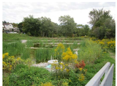
Figure 6.13: Hybrid Wetland – Wet Pond.
