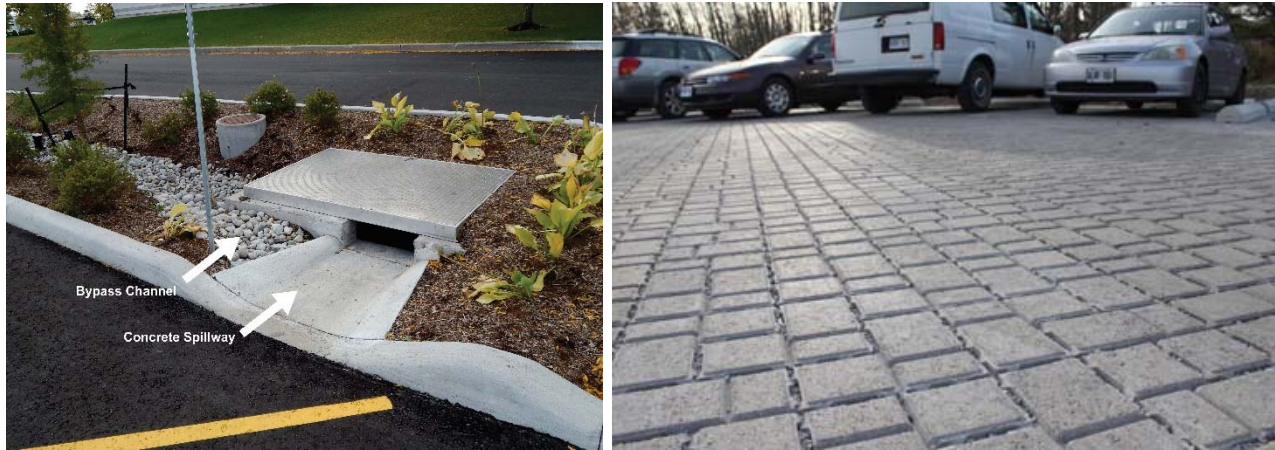
Figure 8.8: Examples of Parking Lot Source Controls
