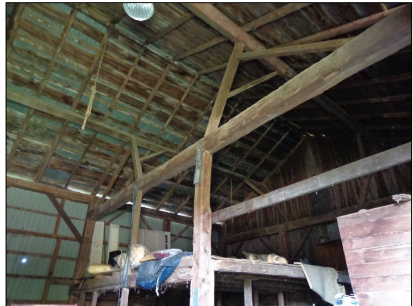
16. Bank Barn Interior; Heavy timber construction with metal roofing and
