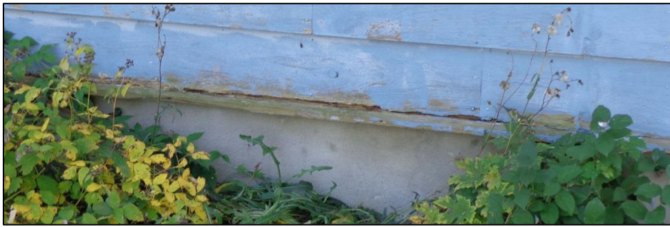
Rot and holes in Wood Siding
