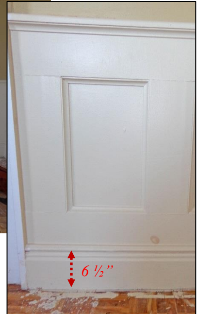
15. Room 2 – Original baseboards & new wainscoting, north wall
