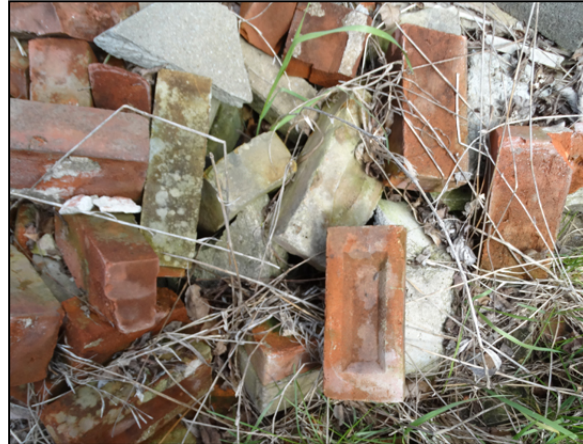
Figure 15: This pile of vintage brick is near the shed and may be the remainders from enclosing the south verandah.
