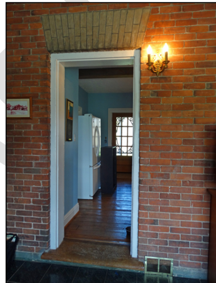
Figure 16: Left: East main entrance into front room, 2017. Right: Looking north from enclosed south verandah, through an exterior wall, into kitchen at northwest, 2017. The corresponding floorboards show a slightly wider and more random tongue and groove flooring in the front room (left), from that of the kitchen (right).
