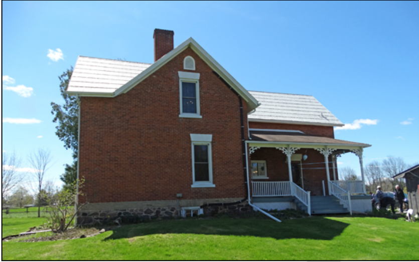
Figure 9: North façade, 2017. The asymmetrical placement of the windows is unusual and may suggest some pre existing section at the front (east).
