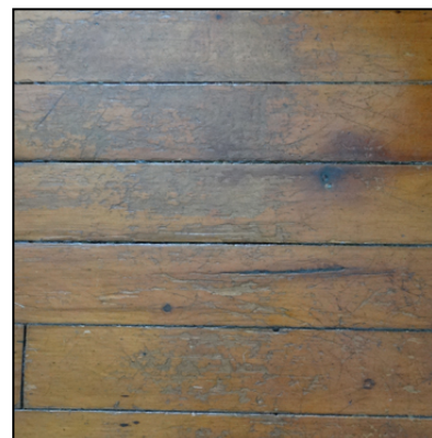
Figure 16: Left: East main entrance into front room, 2017. Right: Looking north from enclosed south verandah, through an exterior wall, into kitchen at northwest, 2017. The corresponding floorboards show a slightly wider and more random tongue and groove flooring in the front room (left), from that of the kitchen (right).
