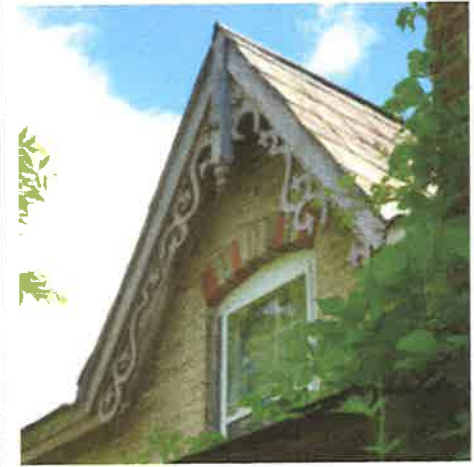
Photos of the Gables around the house. The Kingpost can be seen sitting in front of the bargeboard, unlike the front gable.
