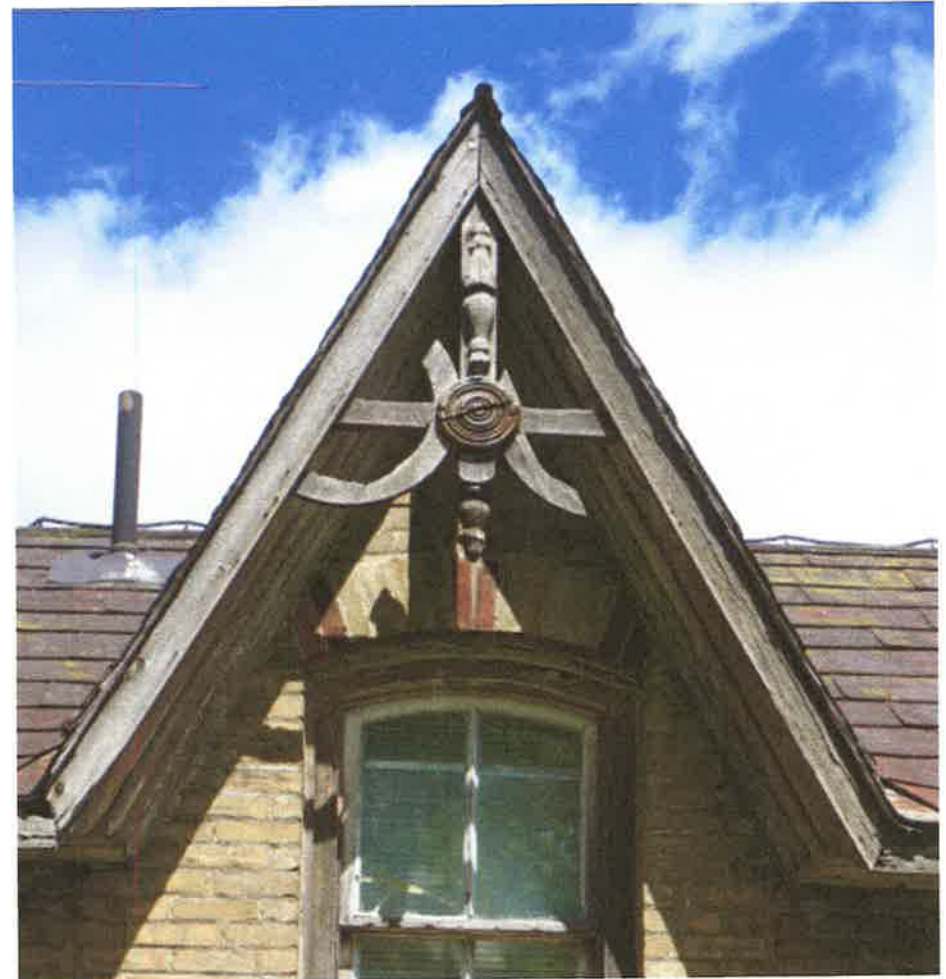
Gable over the front window, featuring a king post design.
