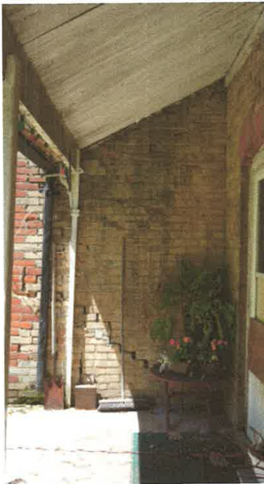
View of the Front Porch. Large wall crack likely due to water damage; freeze/thaw due to lack of downspouts, typical.
