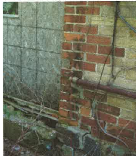
Close-up views of the brick and window sill deterioration.
