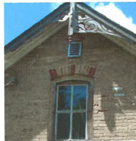
Photos of the Gables around the house. The Kingpost can be seen sitting in front of the bargeboard, unlike the front gable.
