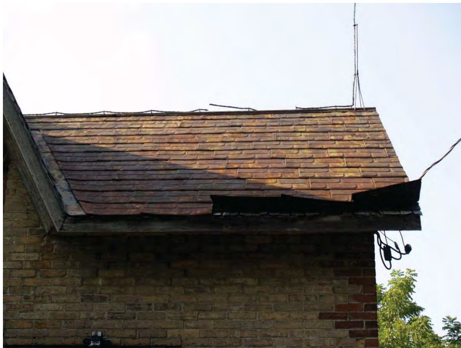
Figure 9: Sheet metal plate roof on south façade.
