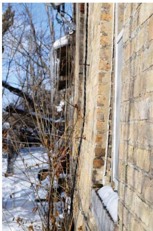
Figure 25: Bend in the west facade wall (February 2018).
