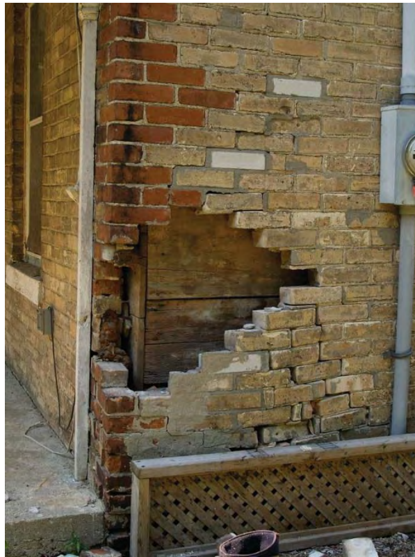
Figure 14: Displaced brick quoins on the southeast corner, exposing the plank-clad balloon frame.
