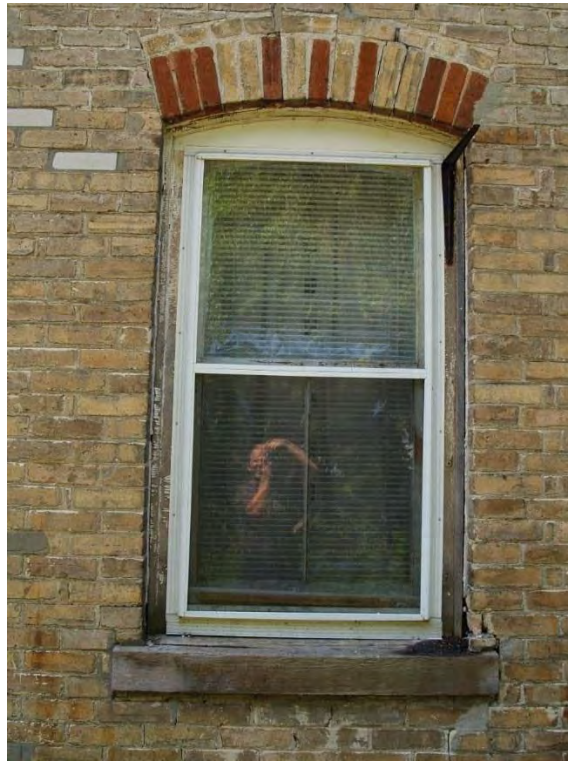
Figure 12: Typical segmental arch head window with dichromatic soldier brick voussoirs and brow or label formed with headers.
