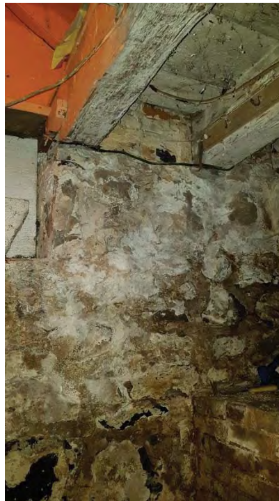
Figure 58: Exposed rubble walls and beams.
