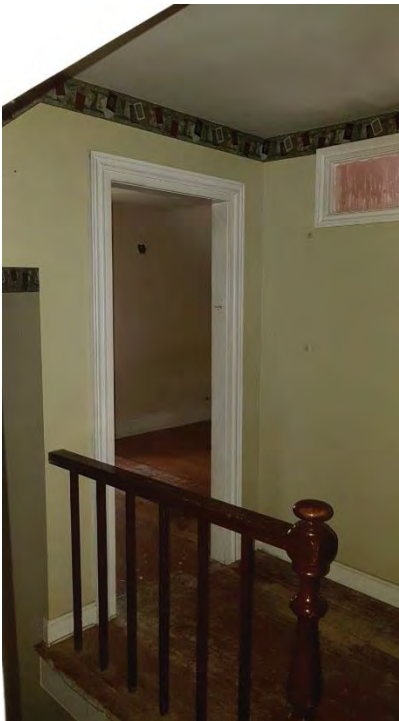
Figure 44: Wood baluster, moulded handrail and plain blusters at second level hallway.
