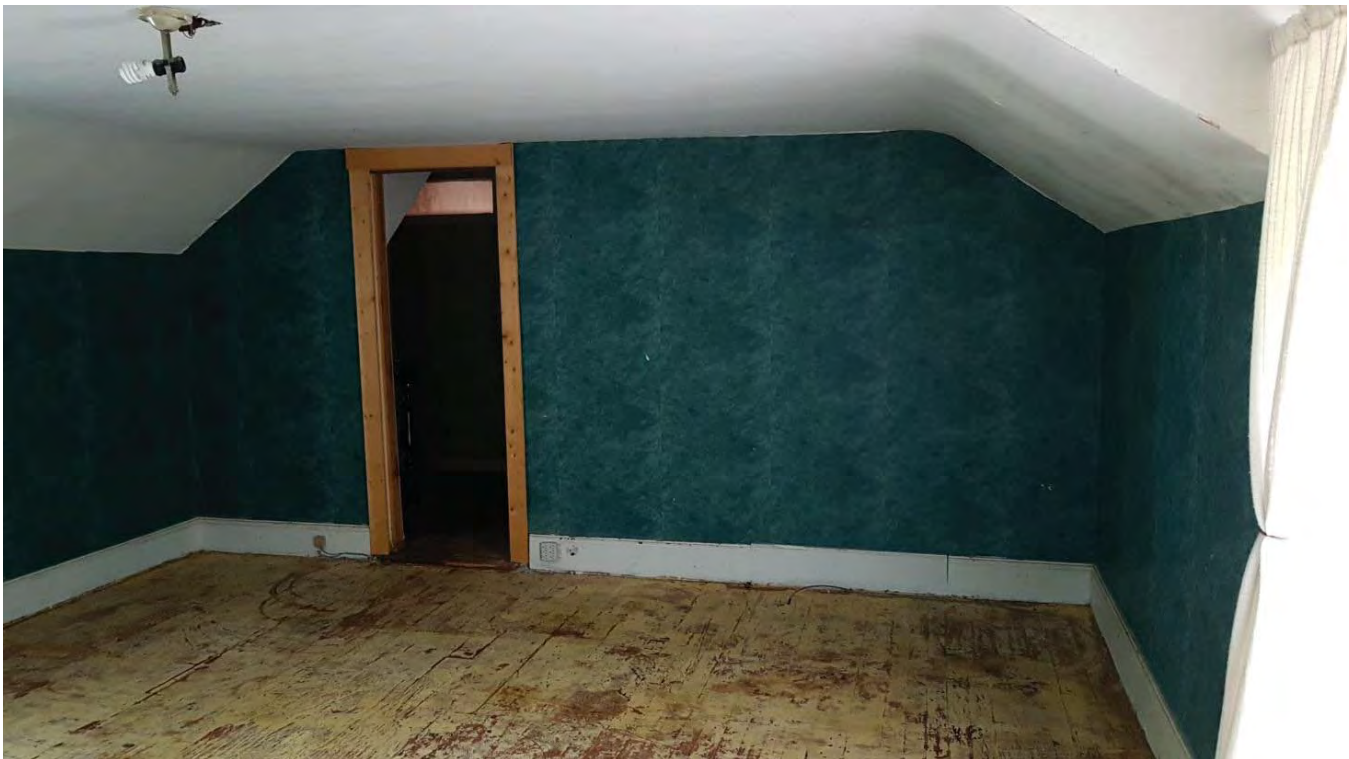
Figure 41: Second level room of the rear wing with 3-inch wide tongue and groove planking.
