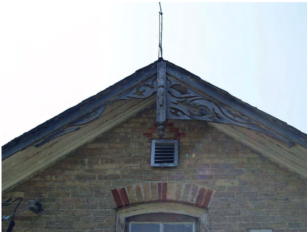
Figure 19: Curvilinear verge board and diamond brick detailing in gable roof.
