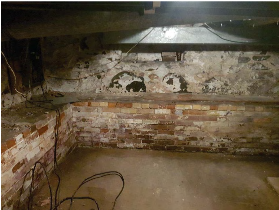
Figure 55: Exposed rubble walls with brick buttress in the basement.
