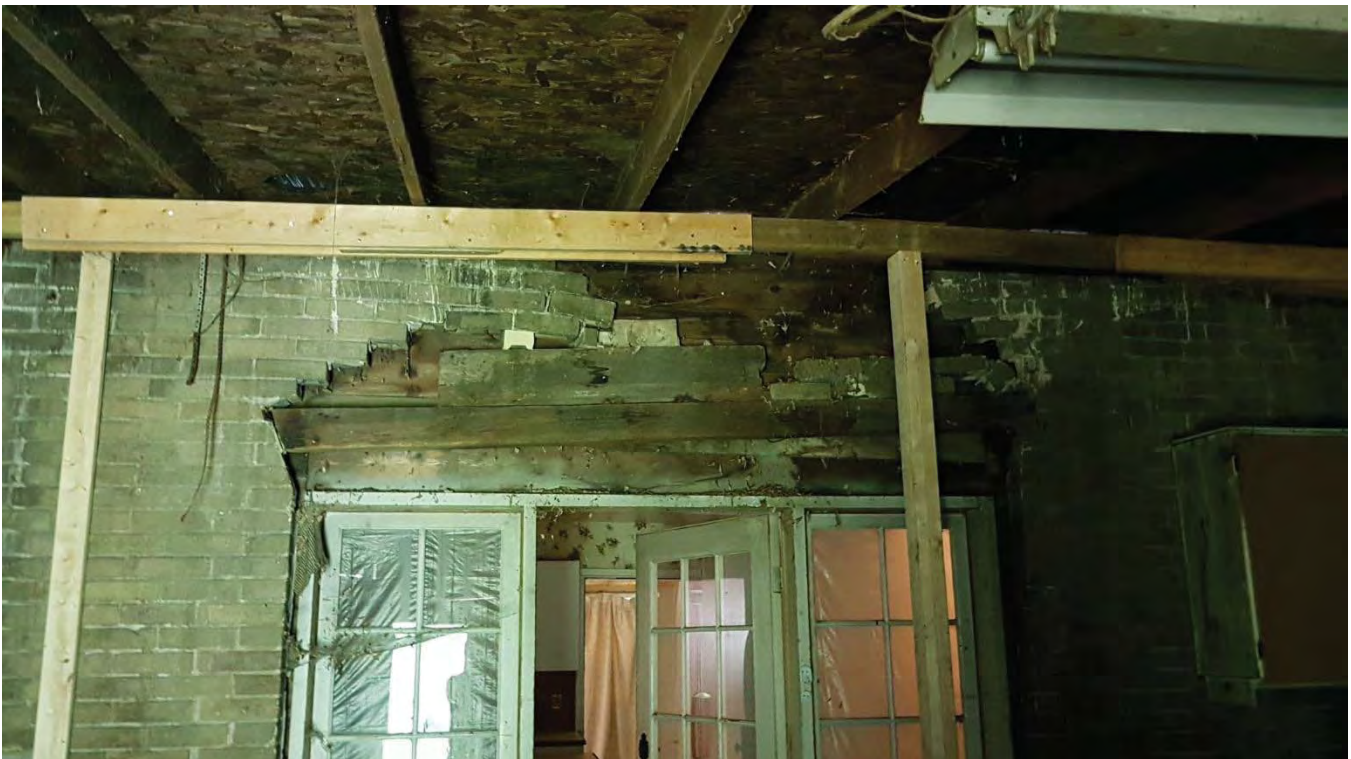
Figure 61: Deteriorating brick in the east lean-to.
