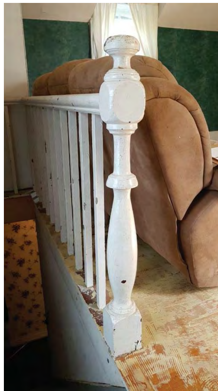
Figure 39: Turned baluster at top of stairs to rear wing.
