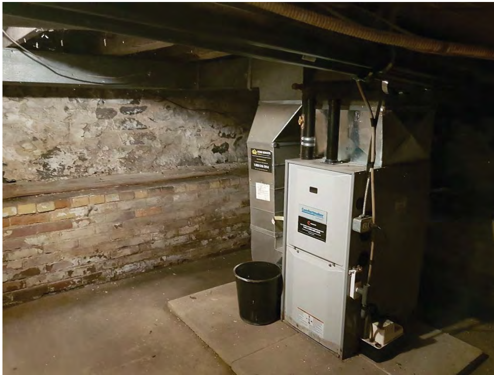
Figure 56: Concrete flooring and rubble walls in the basement.
