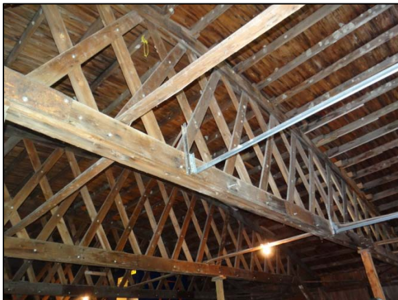
Figure 80: Belfast Truss system within the Warehouse Building.
