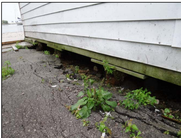
Figure 106: Wood footings beneath the Workshop.
