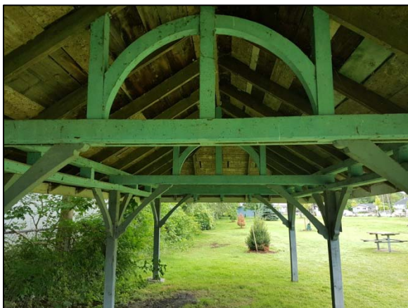
Figure 118: Truss system within the pavilion.
