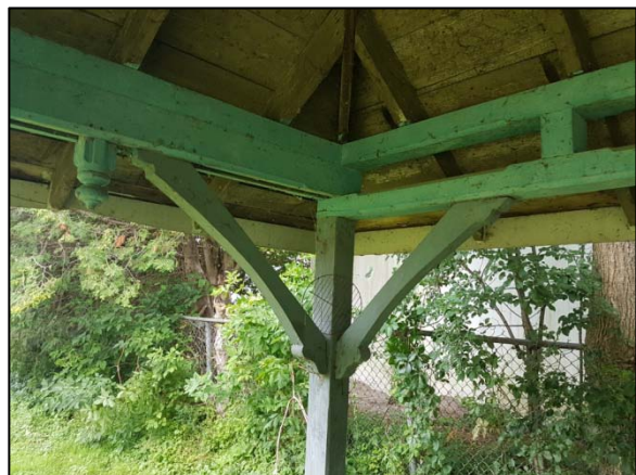
Figure 119: Truss and brace system.
