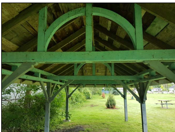
Figure 118: Truss system within the pavilion.
