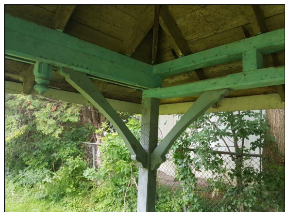
Figure 119: Truss and brace system.
