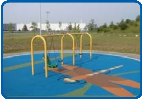
Poured in place rubber surfacing (photo courtesy Scott Belair)
