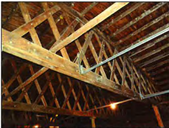
Figure 80: Belfast Truss system within the Warehouse Building.
