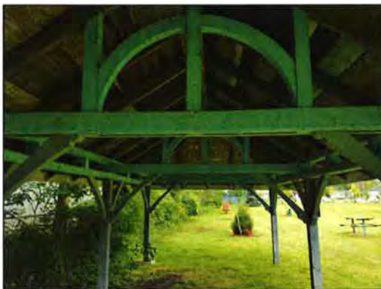
Figure 118: Truss system within the pavilion.
