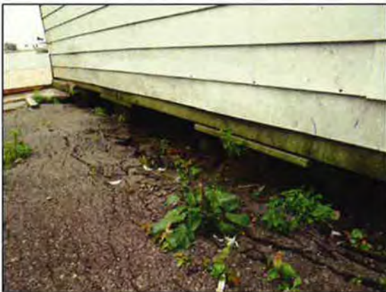
Figure 106: Wood footings beneath the Workshop.
