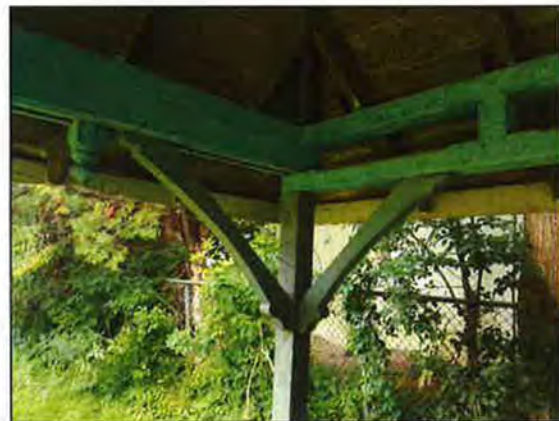
Figure 119: Truss and brace system.
