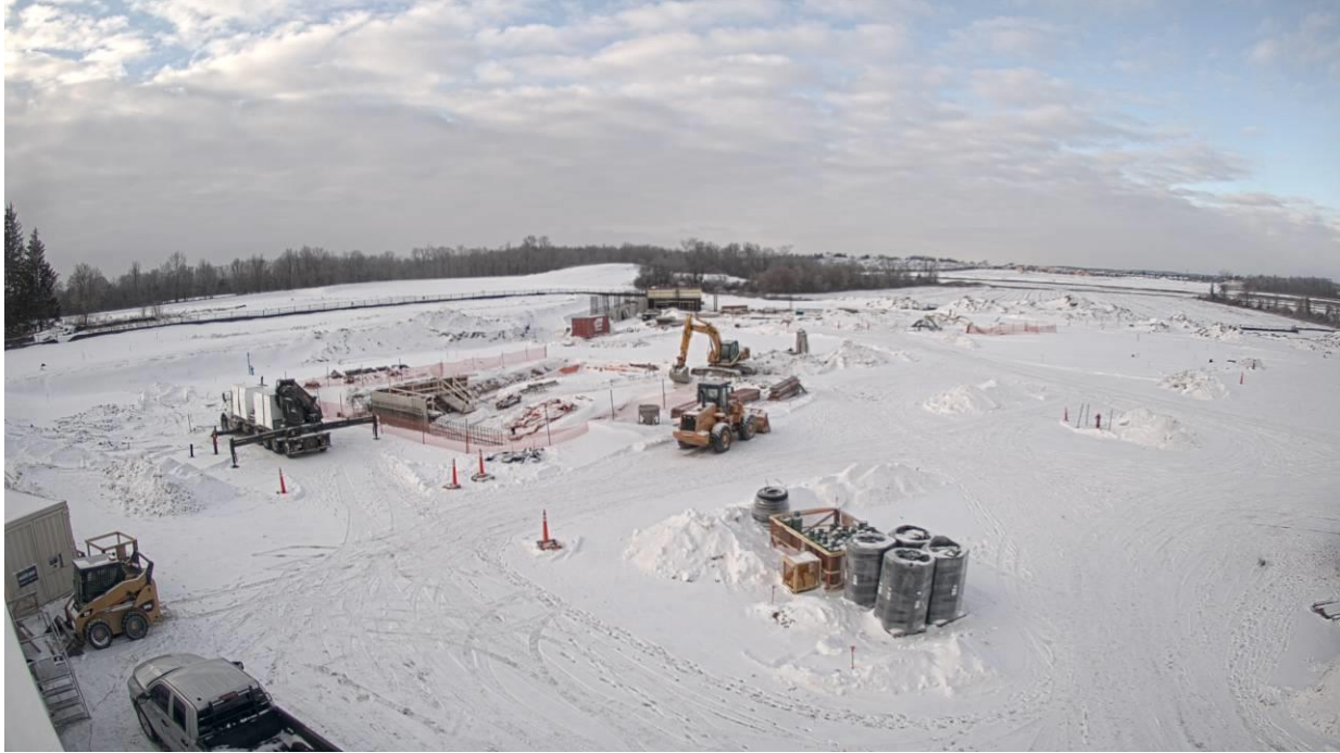
Figure 1 Jan. 26, 2022 Photo from onsite camera
