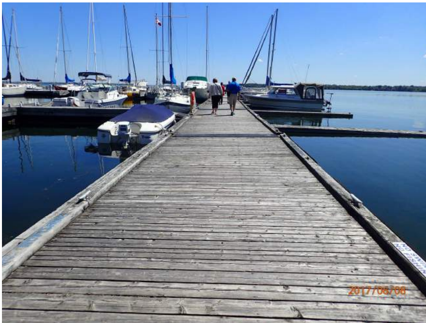
Figure 2.9: Pile supported timber docks at marina.
