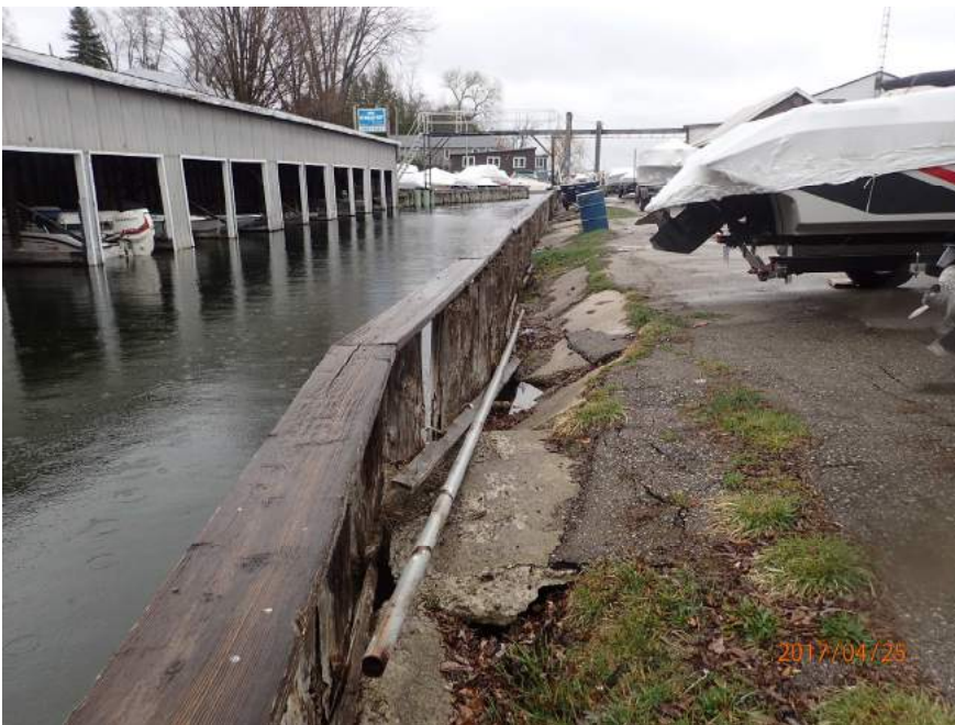
Figure 2.15: View northeast to boathouse with timber wall in a state of disrepair and subsidence behind wall in foreground.
