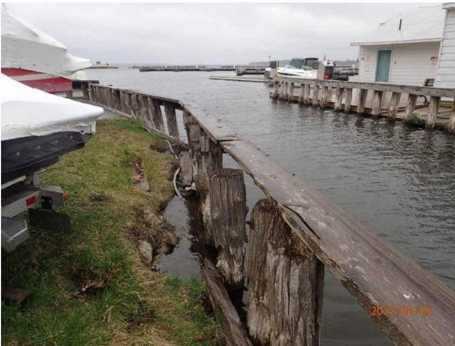
Figure 2.17: Timber wall on north side of canal in state of disrepair.
