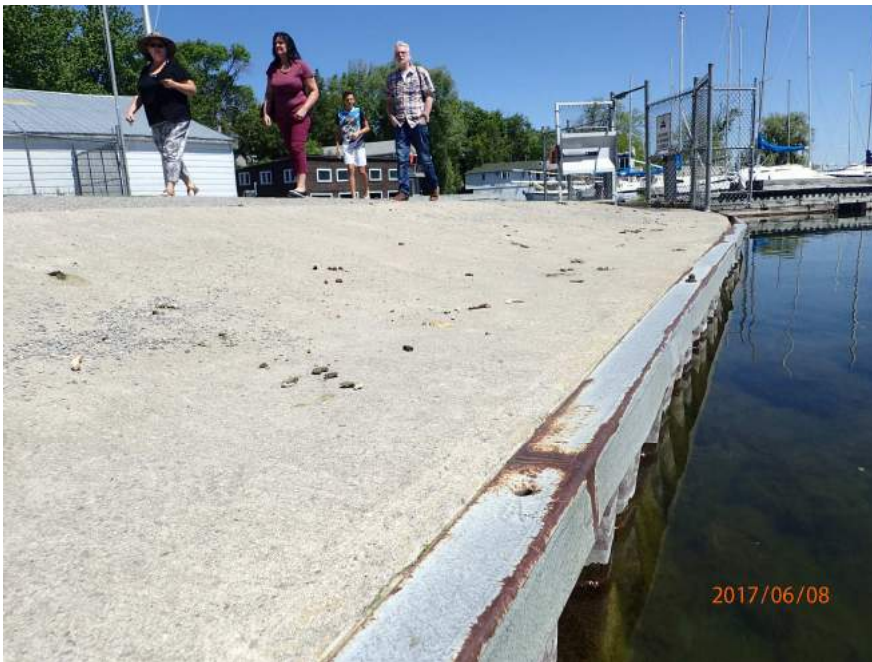
Figure 2.7: Steel sheet pile wall with concrete apron located south of marina.
