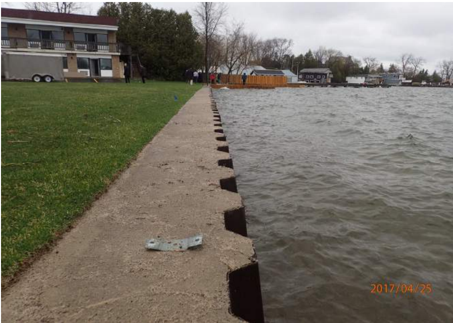
Figure 2.3: View north along Ramada Inn shoreline showing steel sheet pile wall with concrete cap.
