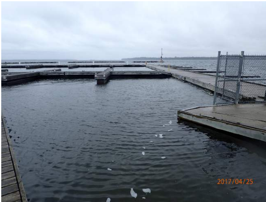
Figure 2.8: Marina with pile supported docks in foreground, rubblemound breakwaters in background.
