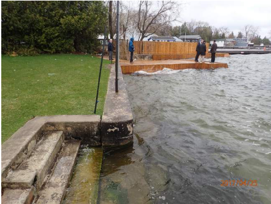
Figure 2.4: North end of Ramada Inn property showing concrete seawall in foreground, wood faced concrete dockwalls in background.
