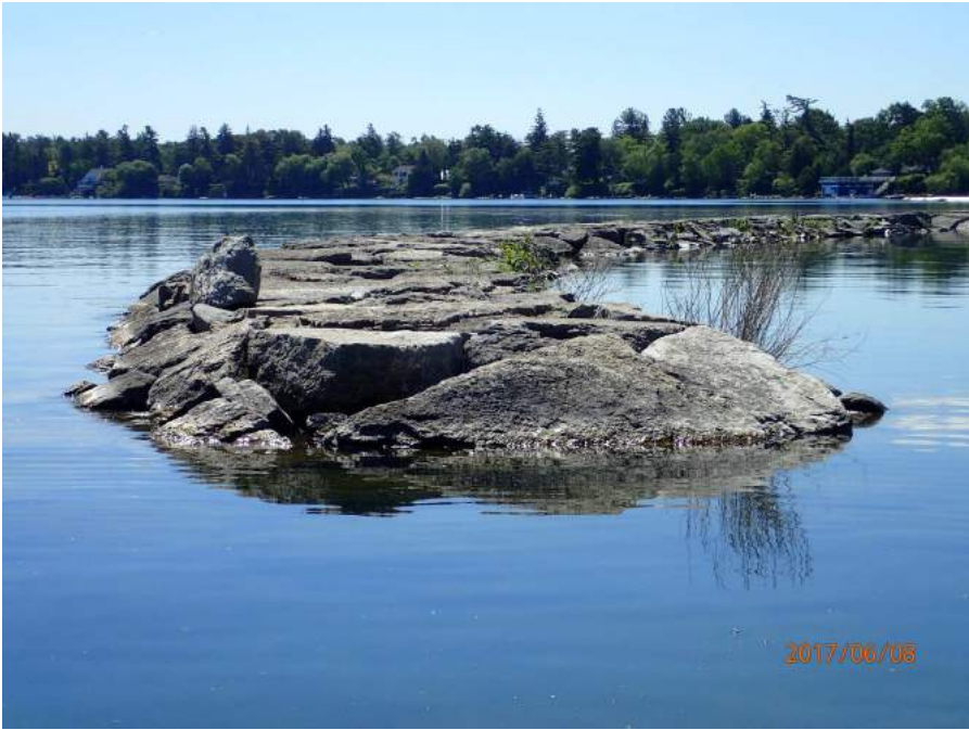
Figure 2.10: Rubblemound breakwater offshore of marina basin, note displaced armourstone.
