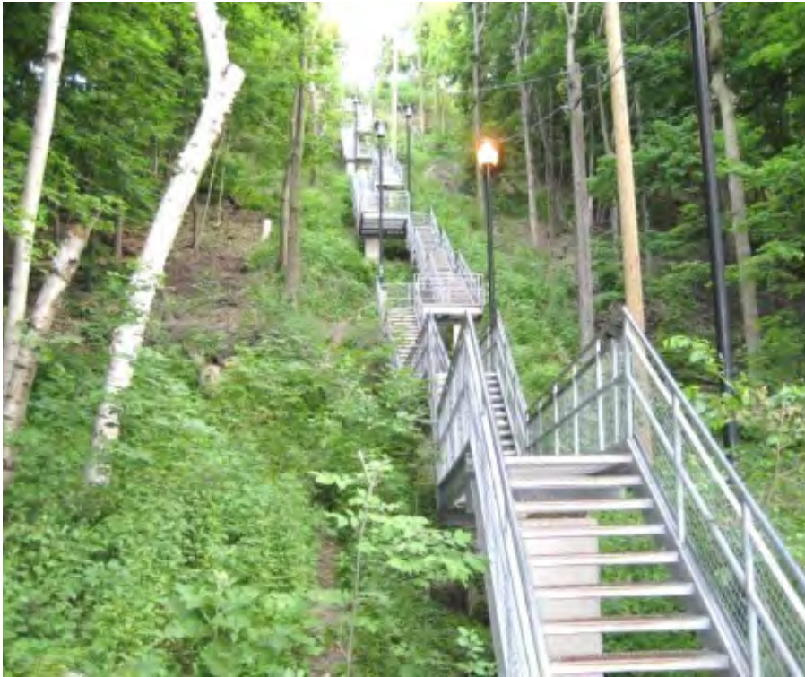
Switchback Example (left) and Woven Metal Stairs, Dundurn Stairs, Hamilton (top)
