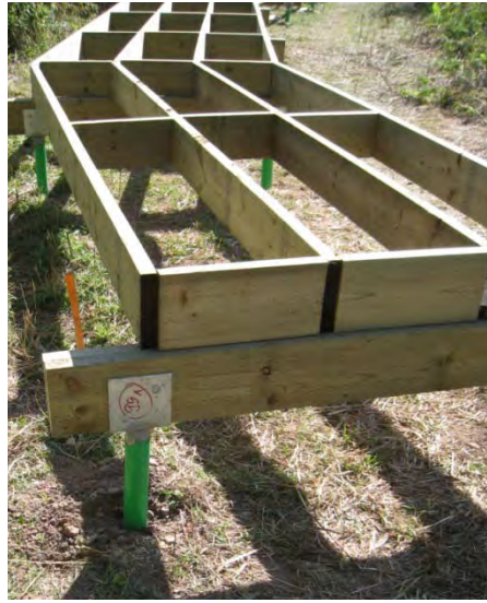
Boardwalk Examples- Hamilton, ON (top) & Boardwalk Foundation on Helical Piles (Halton Hills) (right)
