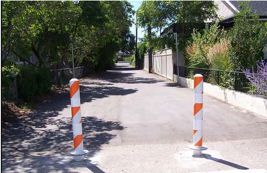
Bollards Implemented at Trail Access Point – Trans Canada Trail, BC
