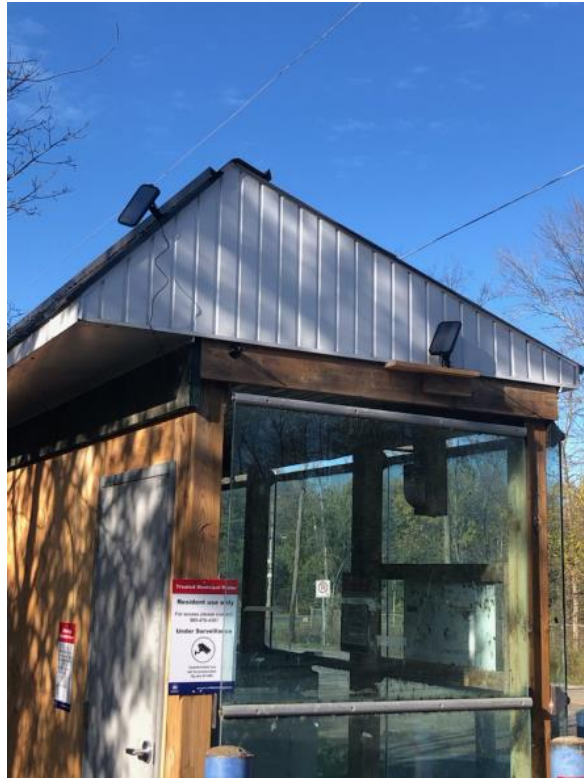
Photo 1 – Black River Road Public Tap with Enclosure
